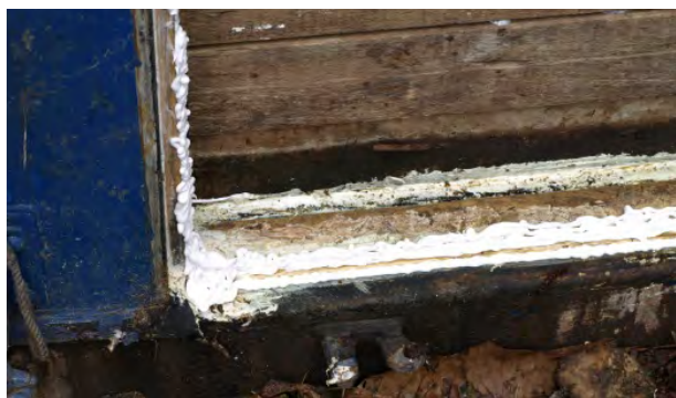
Figure 14: Door prepared to be closed
