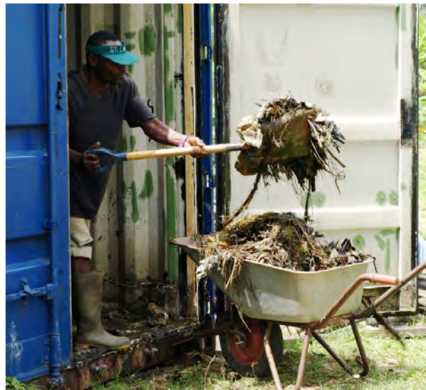
Figure 27: Unloading of the digestate
