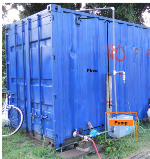
Figure 3: The percolation system with flow direction
