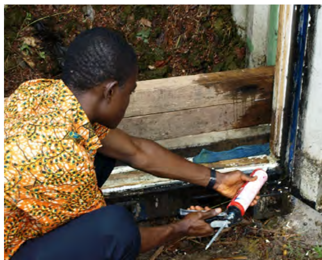
Figure 13: Silicon sealing using a silicon gun
