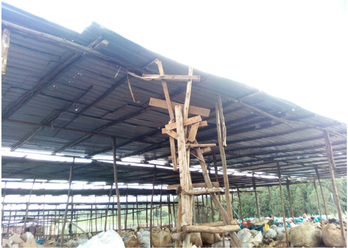
Construction of roof
