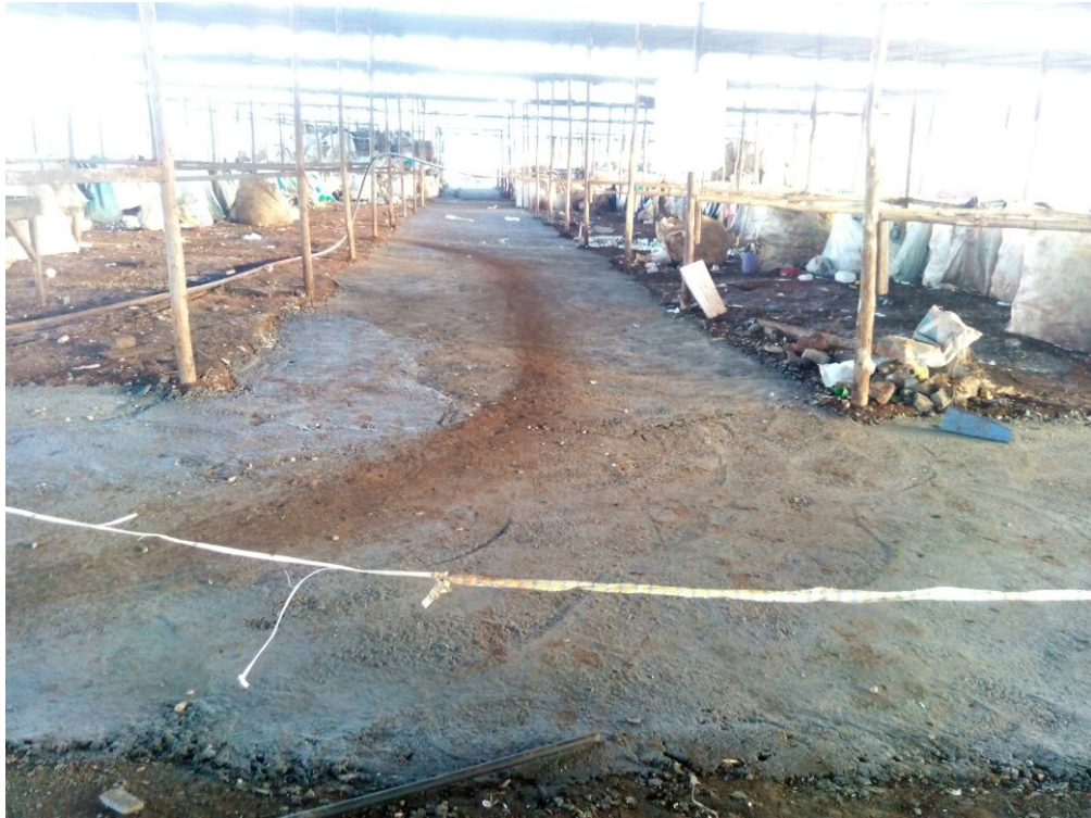
Concreting of floor
