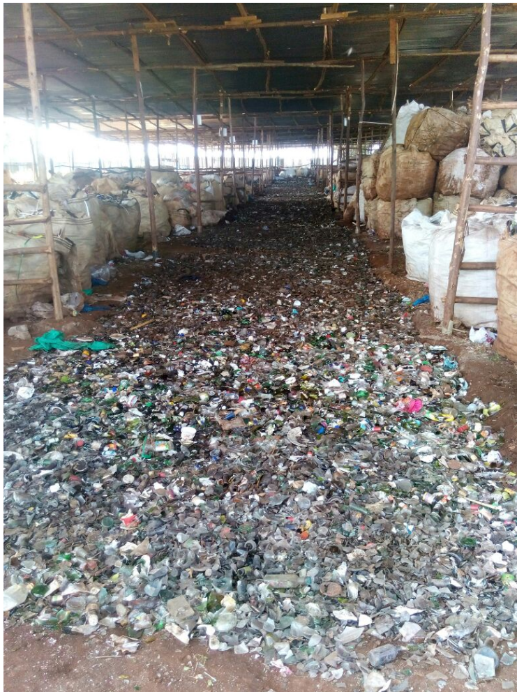
Concreting of corridors using broken bottles as a foundation
