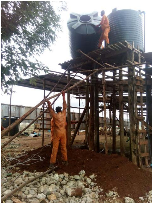
Installation of water tank
