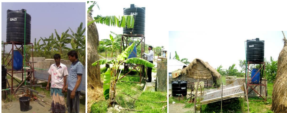
Picture 6: SoWaDis-system with manual treadle-pump at Dhighi, Nasir Samaj, Chargazi, Ramgati, Lakshmpur
