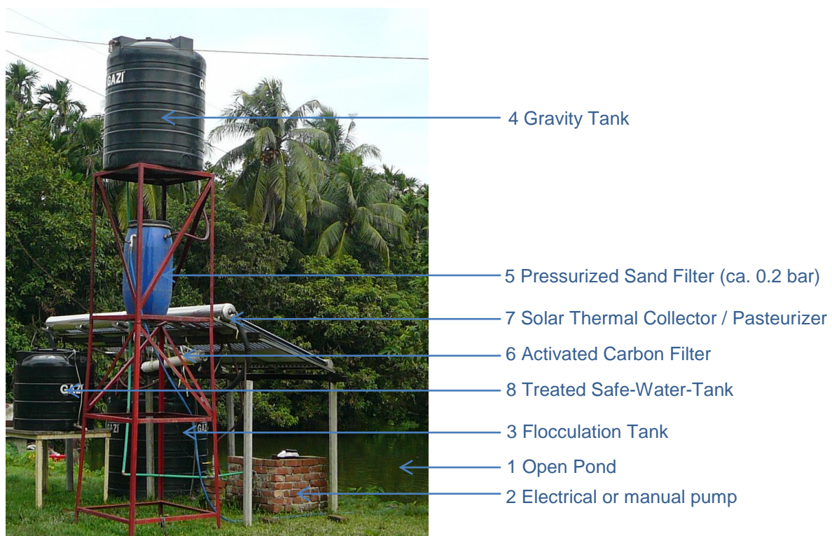
Picture 3: Different components and process stages of the further developed SoWaDis-System 2.0.
