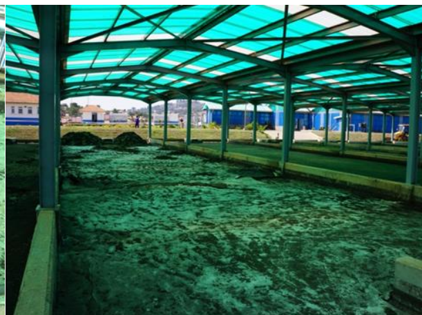
Figure 4: Geotextile on the surface of a drying bed.
