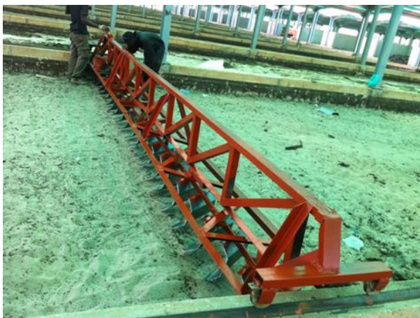
Figure 3: Device turning sludge during on drying beds.
