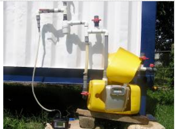
Picture 10. Installation for gas measurements
