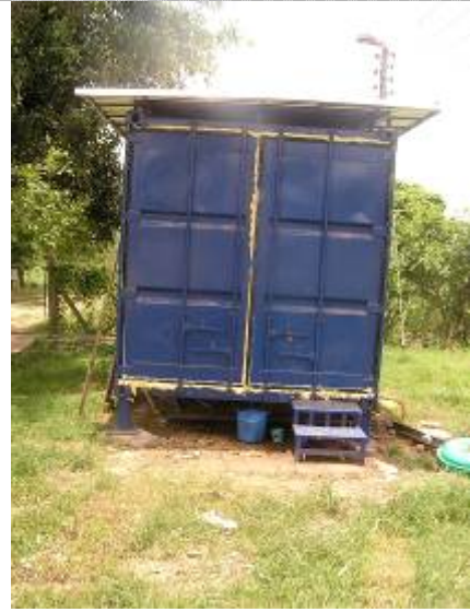
Picture 8. Sealed doors
