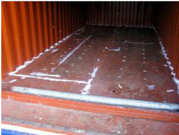
Picture 9. Pipe for percolate collection
