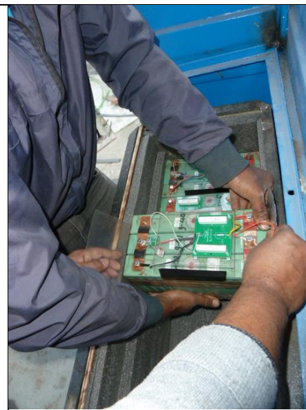
25. Mounting of batteries
