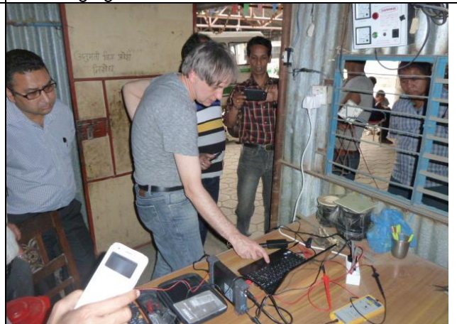
4. Checking the electrical net in a charging station
