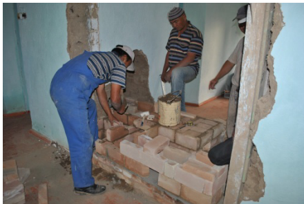
Working process during seminar on energy efficient stoves construction
