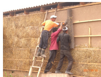
Working process during seminar on house insulation, Jety-Oguz village
