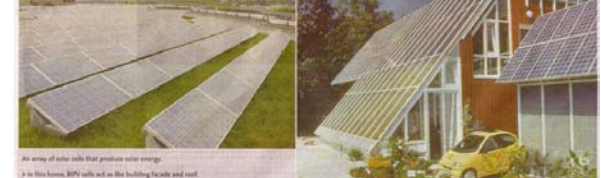
An array of solar cells that produce solar energy. In this house, BIPV cells on the building facade and roof.
