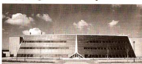
In Europe and Japan, Building Integrated Photovoltaic technology is used in a building facade. Photovoltaic (PV) only integrated into the building shell generates solar energy. PV cells also give a unique architectural look to the building and replace the cost of conventional building material.
