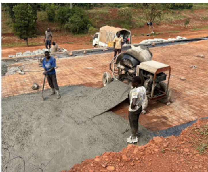
Mafubira Site, pouring concrete foundations for the treatment houses, October 2024
