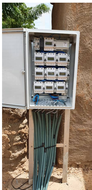
On the left: the process from design to implementation of the Powerhub containing the Power-Blox solar battery systems. On the right the Meterhubs containing the Flexmeters monitoring the consumption of the household connections.
