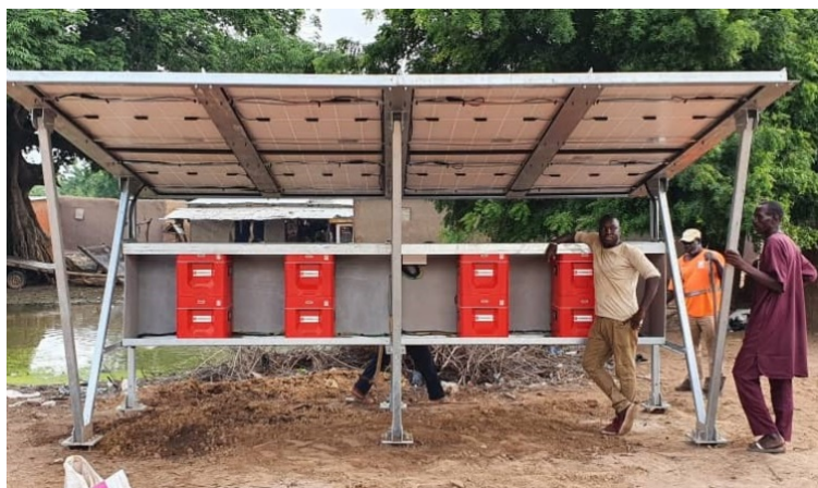
On the left: the process from design to implementation of the Powerhub containing the Power-Blox solar battery systems. On the right the Meterhubs containing the Flexmeters monitoring the consumption of the household connections.
