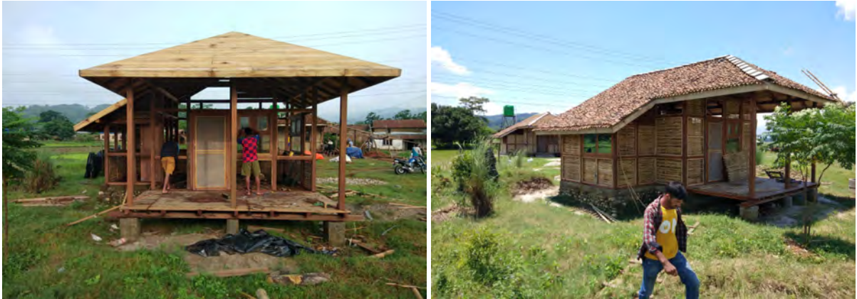
Homestay 2, built independently by community during second lock-down
