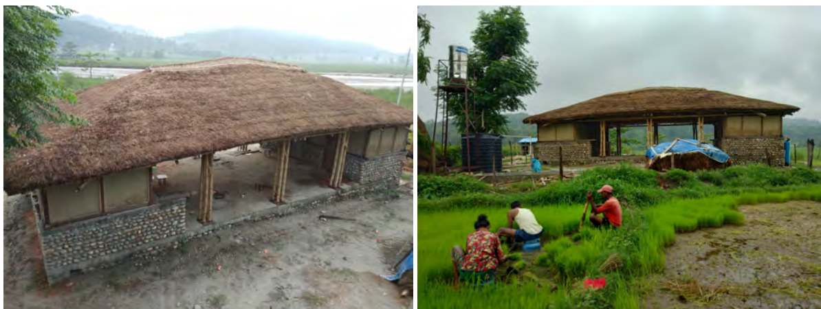
The community hall – with Elephant Grass roof (left); with community planting rice (right)
