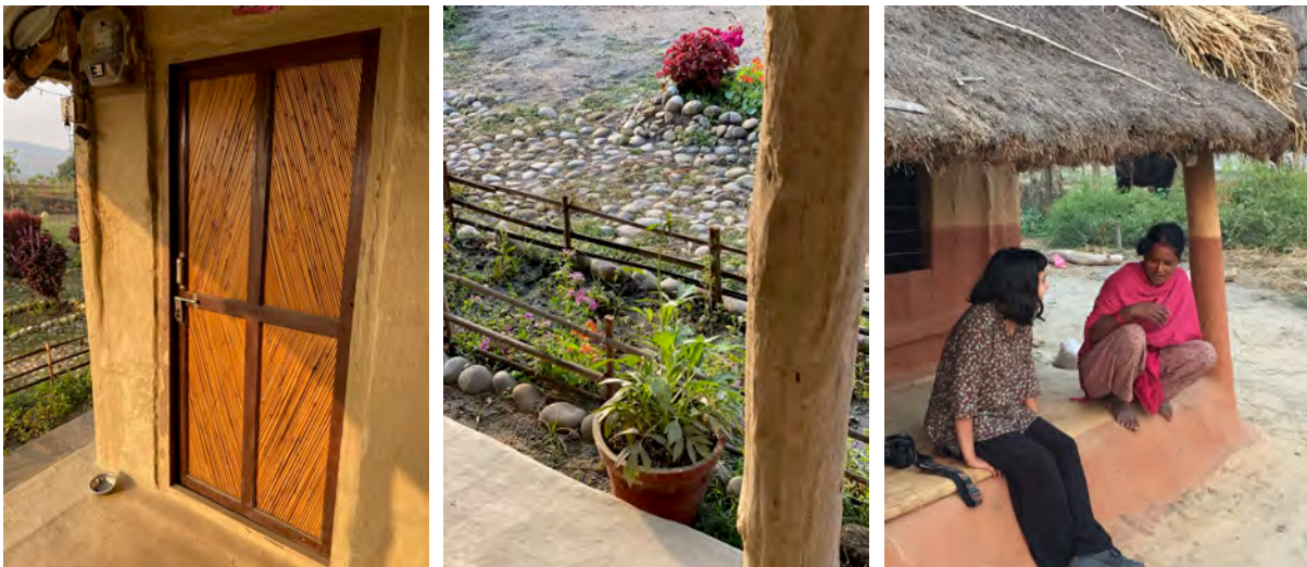
Building back in traditional style: Door and garden deco of local leader Santosh Bot's new house (left, middle), Alisha Adhikari (SMA) chatting with local woman on traditional climate-friendly porch
