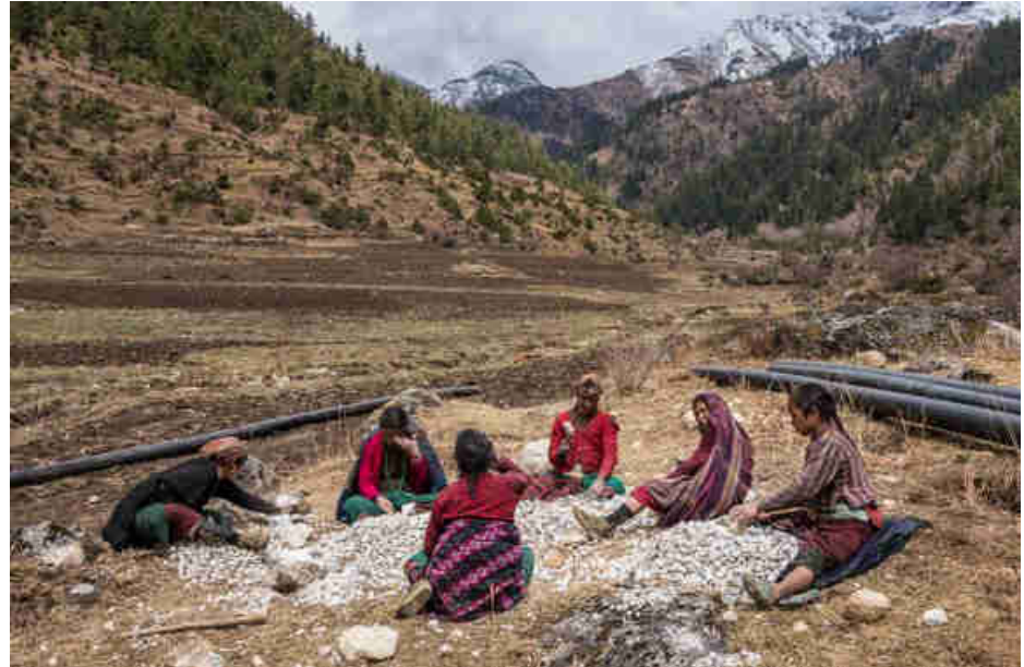
Pic. 88: Women crushing stones with a hammer for gravel for the cement
