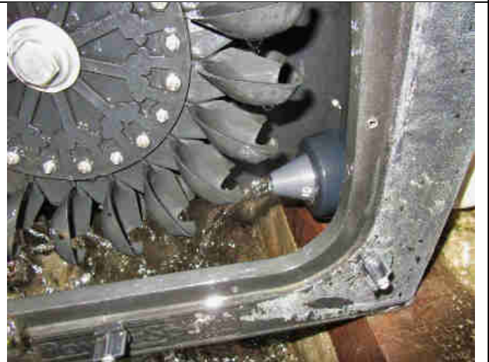
Pic 4: When a turbine is halted for maintenance and cleaning during winter a small stream of water flow has to occur to prevent the water from freezing inside the ball valve keeping it safe
