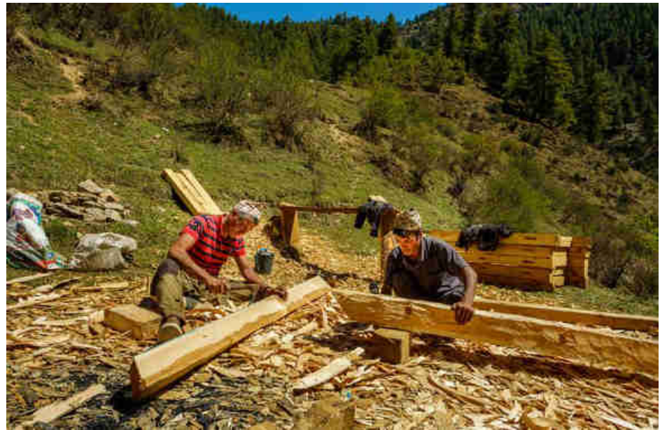
Pic. 110: Carpenters, trained by RIDS, manufacturing the doors and windows
