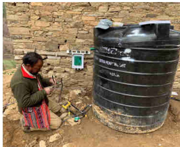
Fig 10: Installation of AC Relay Board and Hot Water Tank for Showers
