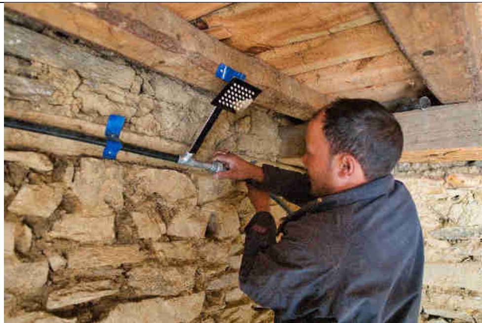
Pic 41: Installation of the shower head in the village based warm/hot shower room
