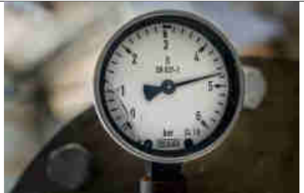
Pic 20: Maximum net head of 47 m (4.7 bars). Based on the village's and power & community house based power demands this pressure is adjusted for power generation
