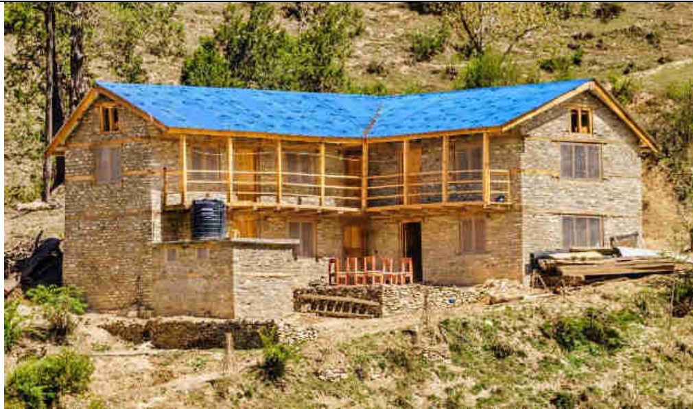
Pic. 34: Power/community house of the modular pico-hydro power plant with the power room, all DC to AC equipment, the battery bank and the AC distribution
