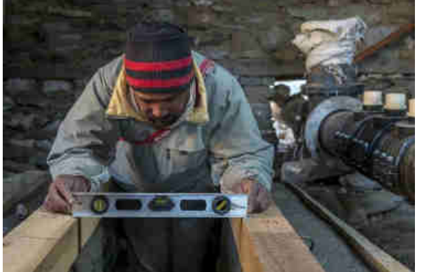
Pics. 55-57: Inside the Pico Hydro Power Plant Turbine house. The last piece (of total 92) of the 5m long HDPE PN6 200 mm diameter penstock is installed and the water canal, to install the 6 Pelton turbines, is built. The 6 PowerSpout Pelton Turbines are installed (screwed on) on top of seasoned hard wood which is resistant to water for 20 years.
