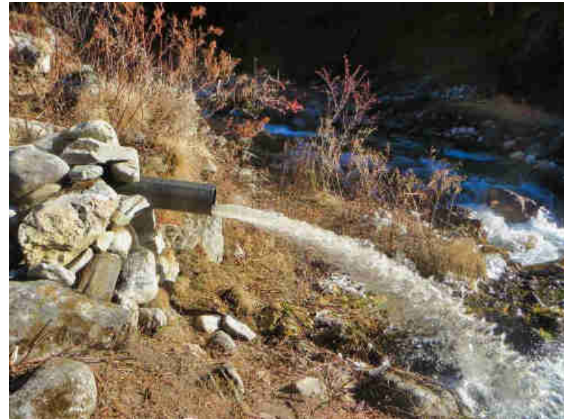
Pic. 8: After the turbines the water is flows back into the river through a 20 m long Ø220mm HDP pipe. In summer this has become an attractive playground for the children, while in winter amazing icicles structures are created.
