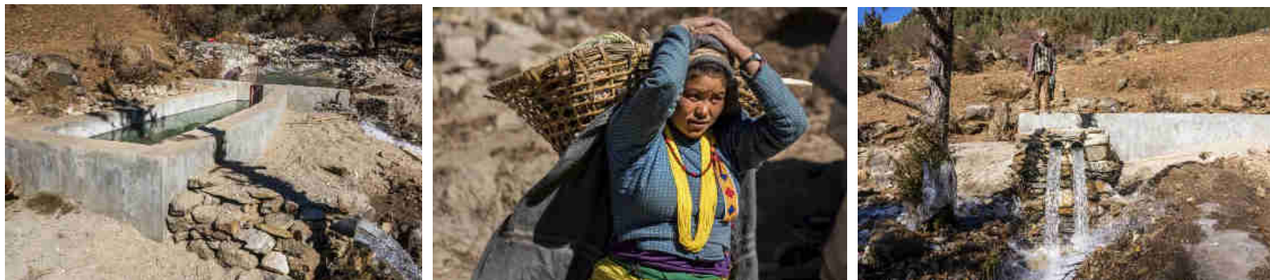
Pics. 91-94: Finished building and operating the sedimentation tank, providing the 6 PowerSpout Pelton turbines with very clean water, without any sand or silt particulates. That will increase the life expectancy of the turbines significantly.
