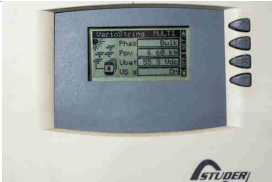
Pic 19: 6.6 kW maximum power generation of all 6 turbines a 47 m, ~ 20 L/sec, resulting in an overall ~72% Power Conversion Efficiency (in AC) in the village
