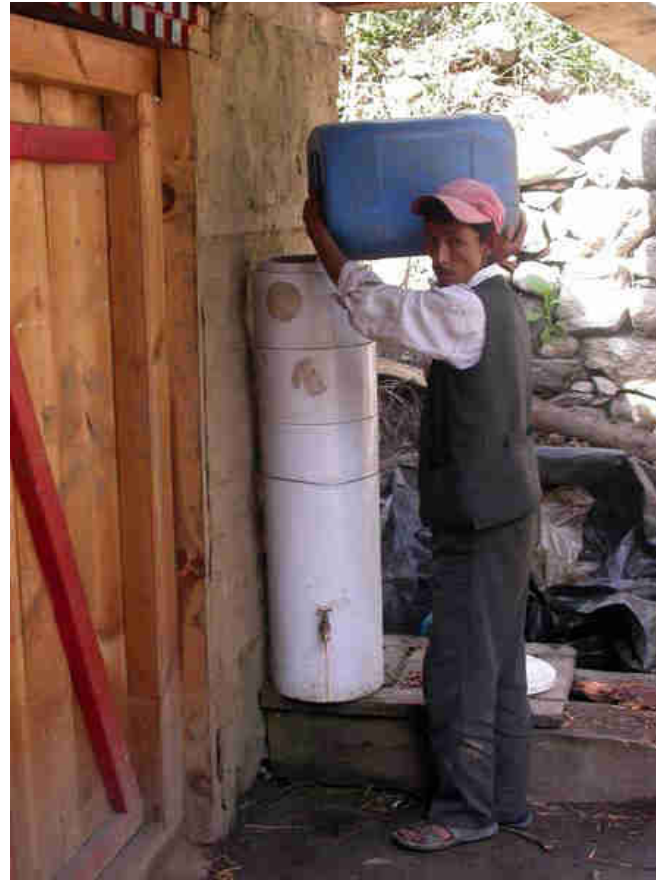
Fig.16: A restaurant owner from another village is filling the slow sand water filter in the morning to be ready when traveler pass by his restaurant and stop for a snack or something to eat. As additional service he can now provide with the SSWF clean drinking water and thus makes sure that the travelers stopping at his restaurant, remain health.
