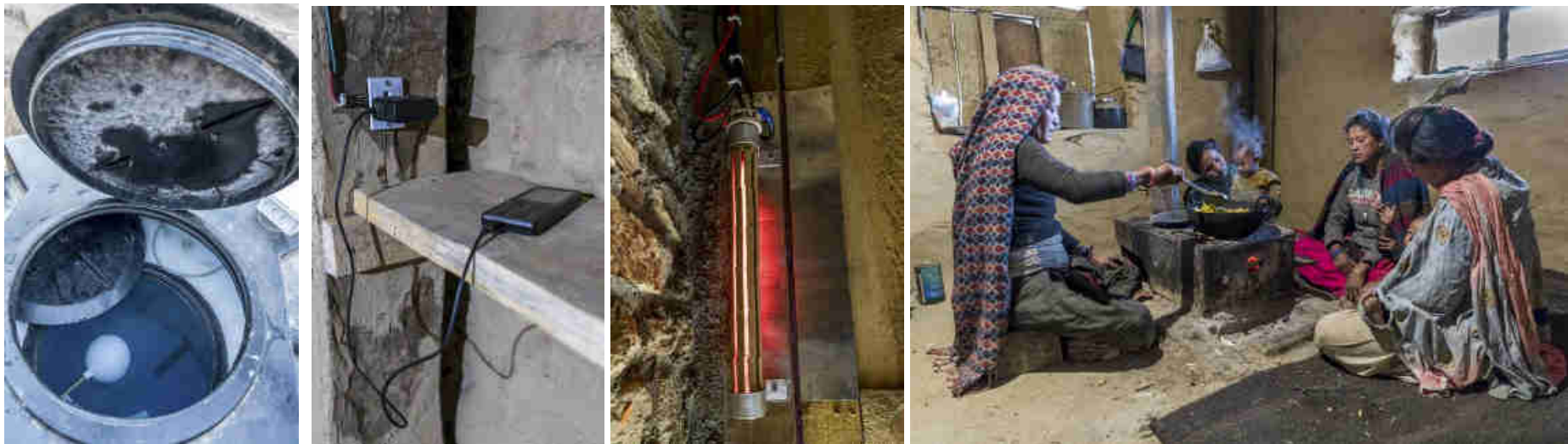
Pics. 128-130: Different users and “smart dump loads”. Left: Warm water heating bathing system (inside 60 °C water with the inside drum lid with ice as the night temperature was around -5 to -8 °C). 2 nd to left: charging of a mobil phone in one of the Mohari family homes. 3 rd from left: Resistor (48VDC) room heater in the power/community house office. Right: Cooking with the RIDS developed smokeless metal stove and a LED light (3 watt) in the kitchen.
