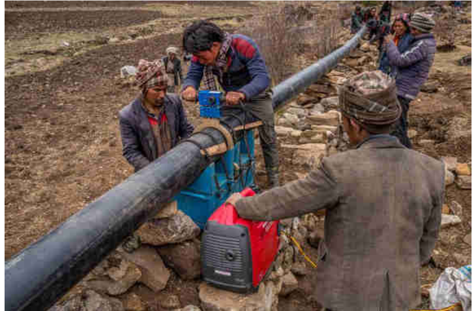
Pic. 36: The metal heating plate is heated with the petrol generator up to 220° C
