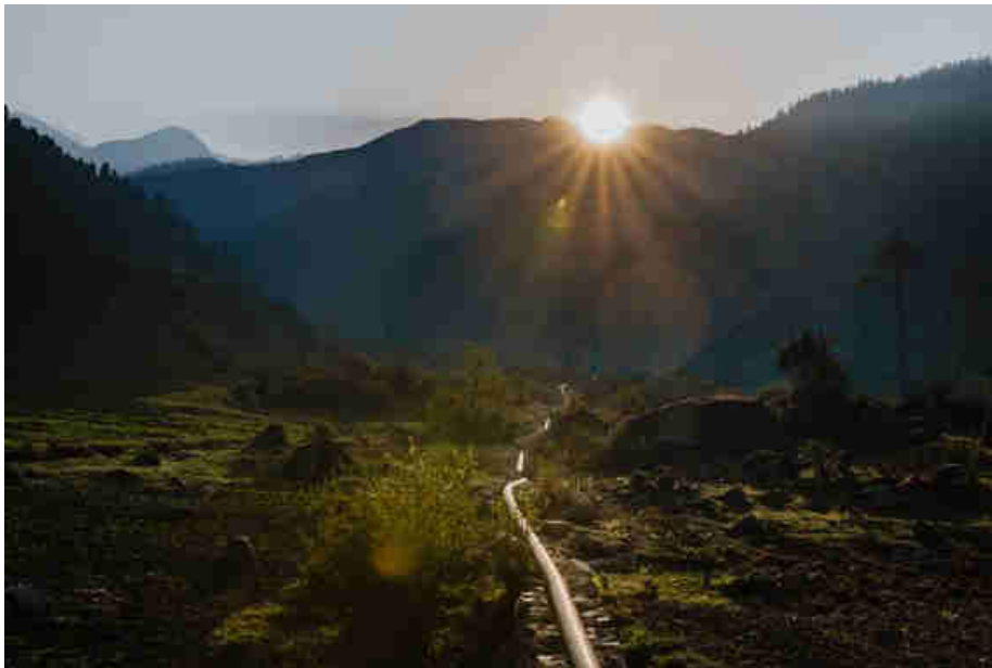
Pic. 73: Sunrise over the modular pico-hydro power penstock pipeline
