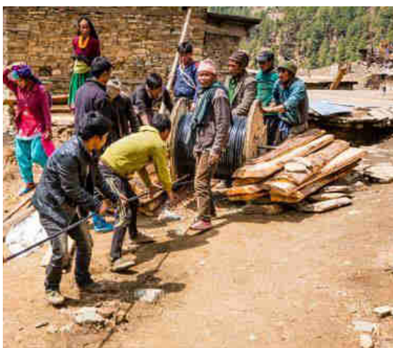
Fig 7: Unwinding Armored Transmission Cable from the Spool
