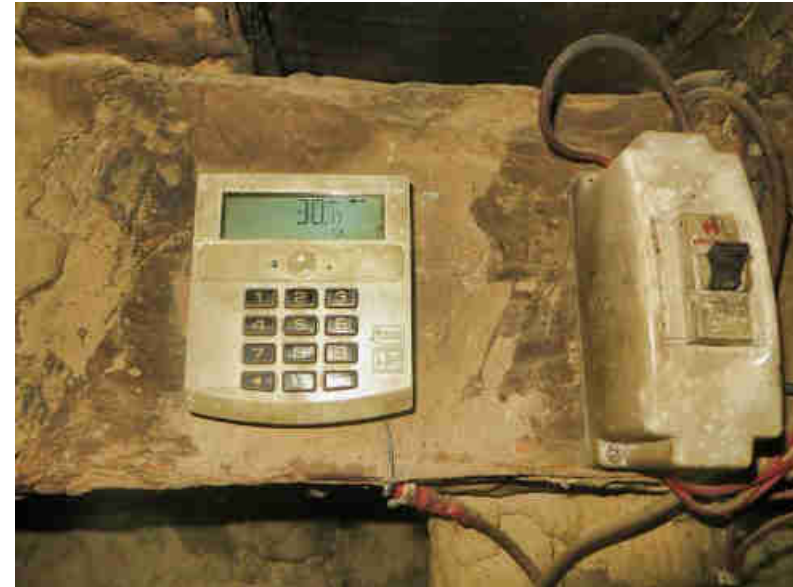
Pic. 24: The smart meter displays the electricity units left (here 30.7 kWh).
