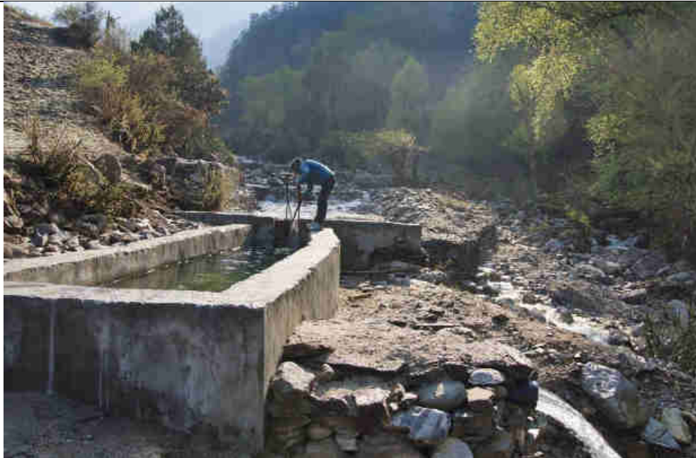
Pic 23: Daily cleaning of the sedimentation tank at the intake
