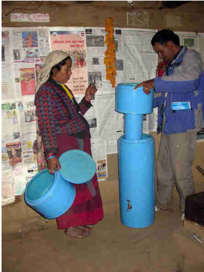
Fig. 15: RIDS-Nepal staff instructing a lady from Mohari, how to install the slow sand water filter inside her home and how to fill it with the sand she collected from the nearby river.
