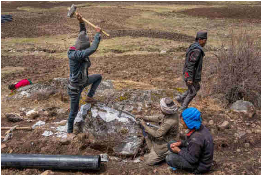
Pic. 17: Clearing the HDPE penstock pipeline path from large rocks
