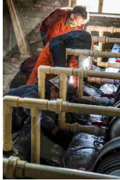
Pics. 70-72: 2" PVC piping installation to connect all the 6 Pelton turbines to the HDPE penstock.
