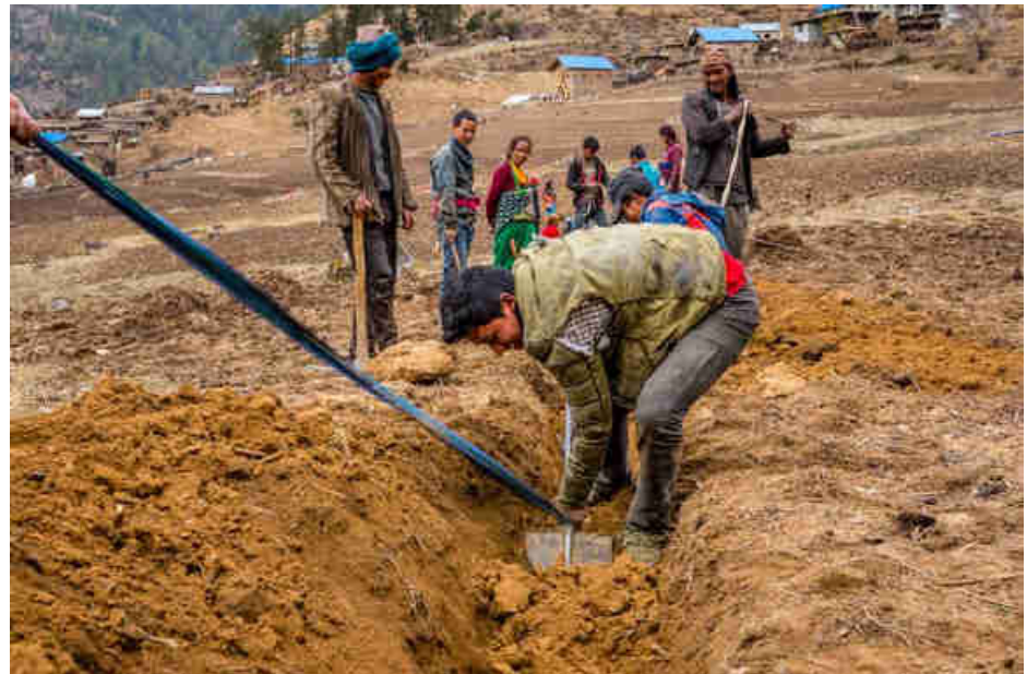
Pic. 22: Digging the canal for the underground power and communication cables
