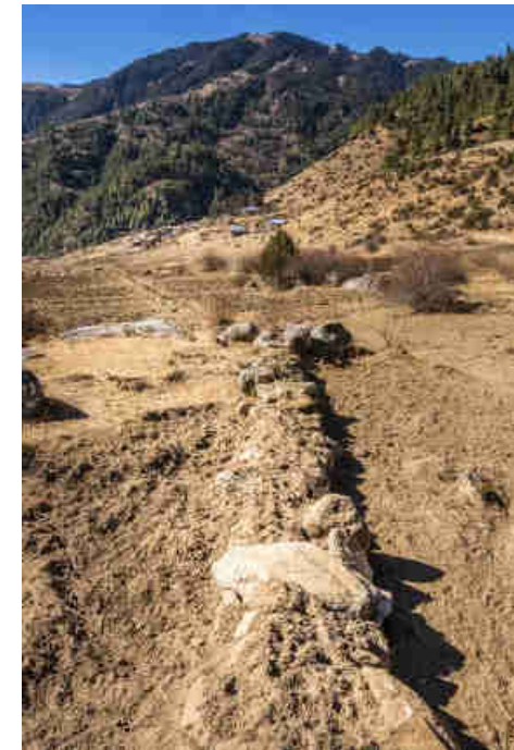
Pics. 18-20: Covered, protected 460 m long, 50 m head, HDPE penstock pipe which carries 24 liter water per second to power the 6 PowerSpout Pelton Turbines.
