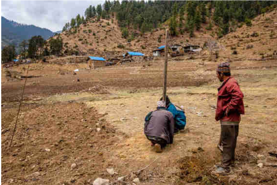
Pic. 11: Surveying underground electrical cable from the turbines to the village
