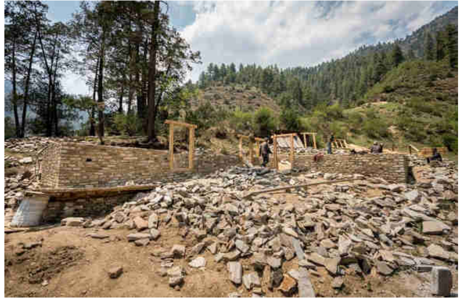
Pic. 116: Building the ground walls of the power house stone walls
