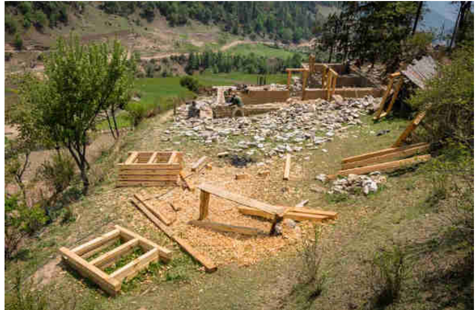
Pic. 118: Power house stone walls and wooden doors and windows
