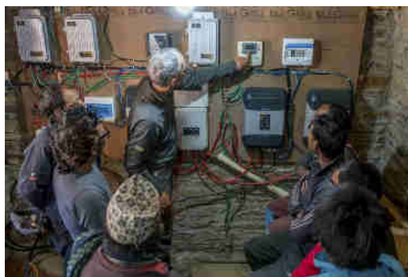
Pics. 110-112: Training of the RIDS staff and operators in the use of all the equipment in the power room by Mr. Mark Staumbaugh. In turn, the RIDS staff is training the local Mohari operators and village elders in understanding what all the pieces of equipment mean and indicate of the Modular Pico-Hydro power plant.
