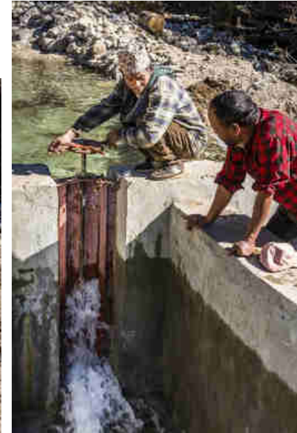
Pics. 82-84: RIDS staff training the two local operators, Aitaram and Hiralal, how to operate and maintain the sluice gate valve of the sedimentation tank.
