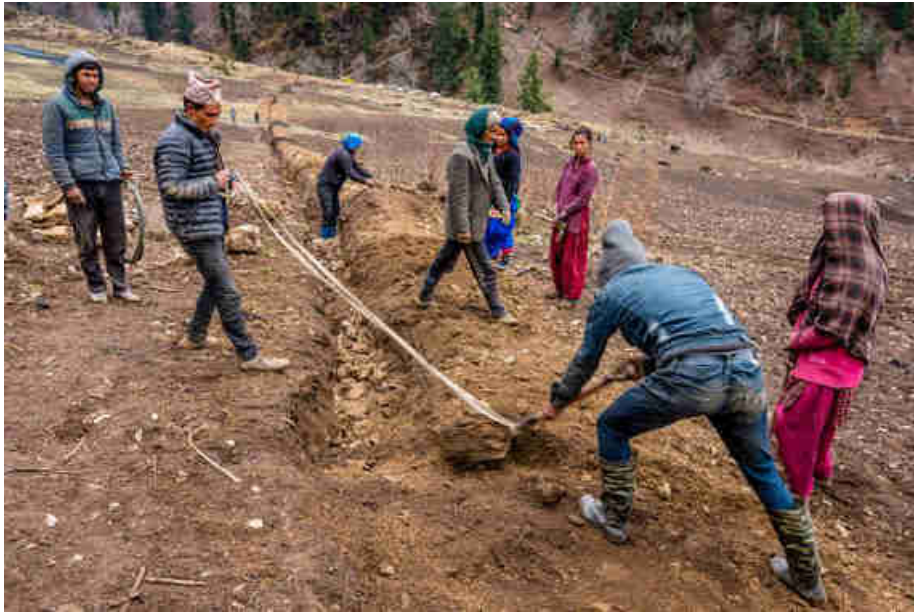
Pic. 33: Covering the power and communication cables with soil for protection
