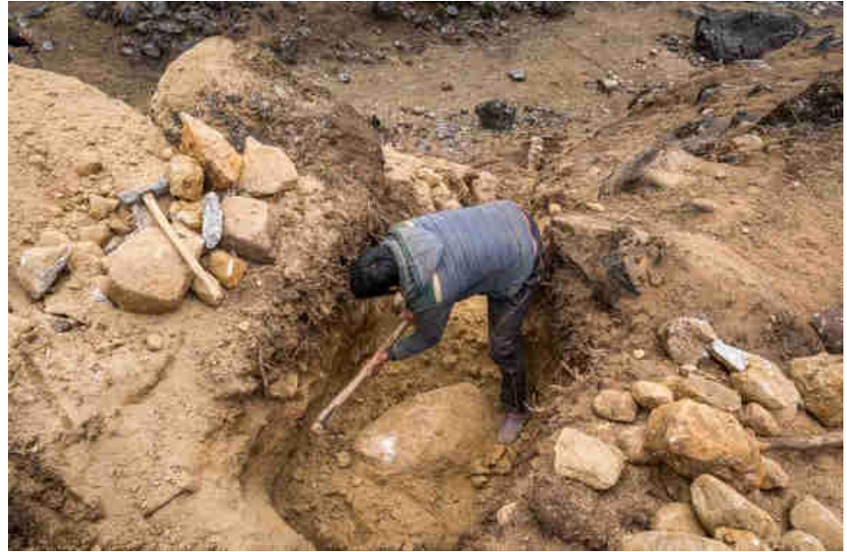
Pic. 16: Clearing the HDPE penstock pipeline path from large rocks
