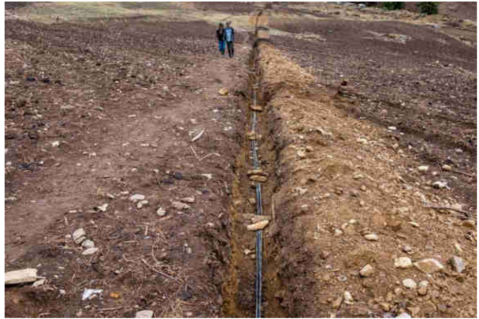
Pic. 30: Layed copper power cable and communication cable before burying them
