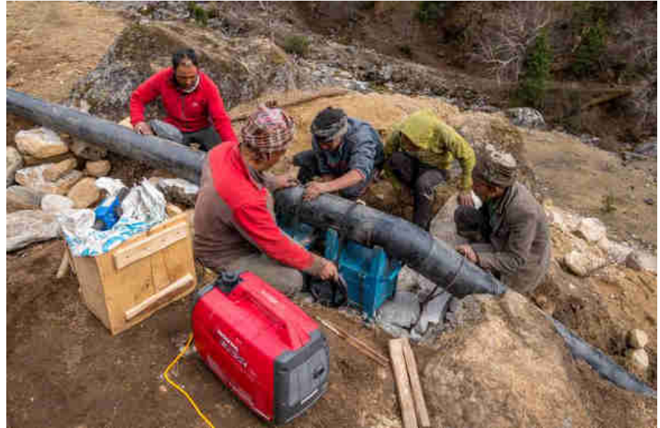
Pic. 44: To weld on the 45° elbow HDPE has been particular a challenge
