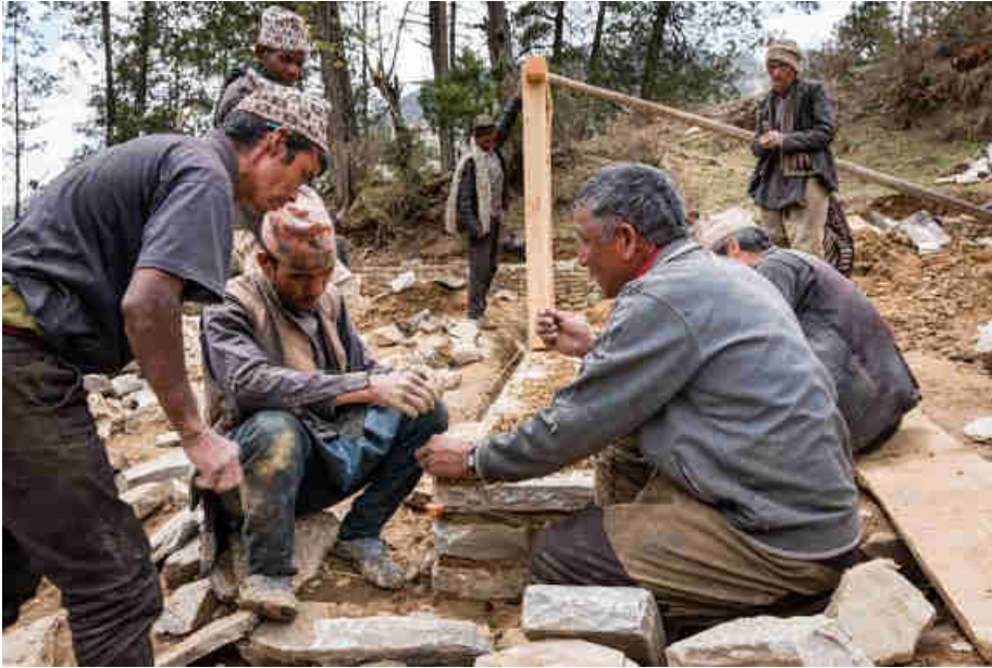
Pic. 103: Building the ground walls of the power house
