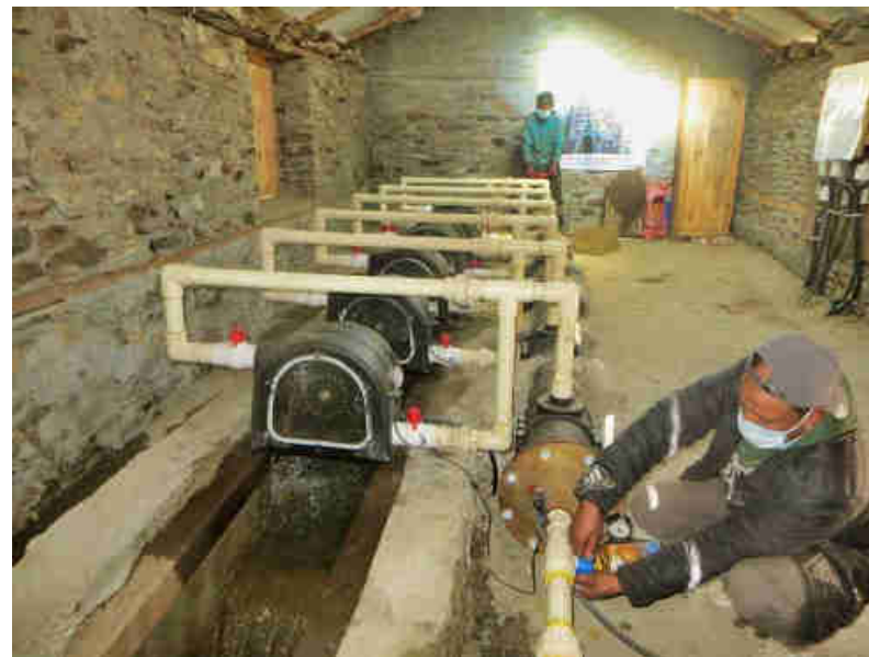
Pic. 10: RIDS-Nepal staff Mansingh cleaning the drainage valve from any leftover sand and small debris which made it into the penstock.
