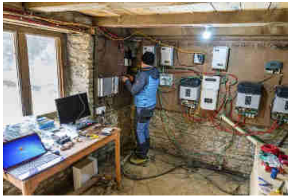
Pics. 95-97: Building the wooden box for the 200Ah 48 VDC battery bank for the Power room. Inside the power room, installing the various power electronic equipments such as the inverters, charge controllers, computer, switches and security systems.
