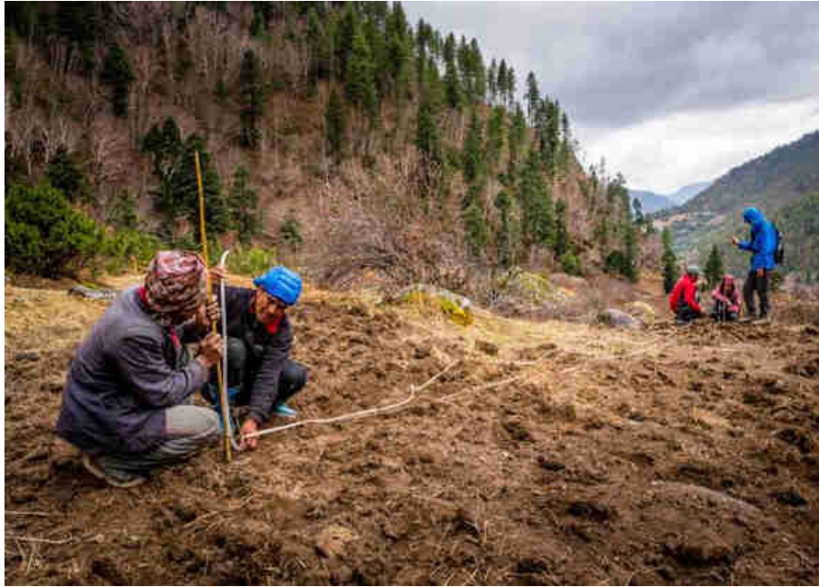
Pic 2: The penstock pipe line is surveyed several times
