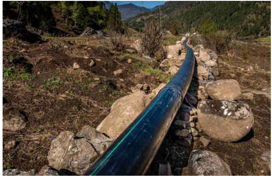
Pic. 46: Welded 200mm diameter HDPE penstock ready for the pressure test
