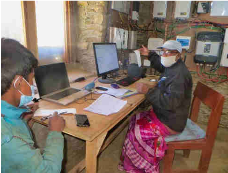
Pic. 21: Monthly electricity token is generated through the PC via specially installed Internet line for each household after pre-paying the monthly fee.
