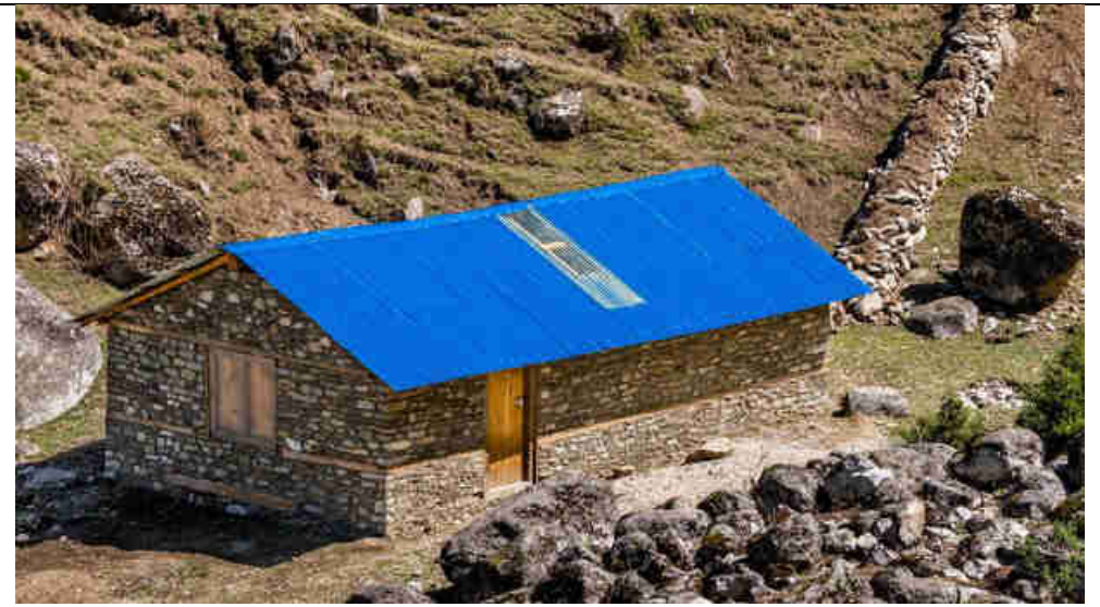
Pic 4: Turbine house of the modular pico-hydro power plant with the 6 PowerSpout Pelton turbines. 47 m Net Head, ~20 L/sec flow, 6.6 kW power generation = ~ 72% eff.
