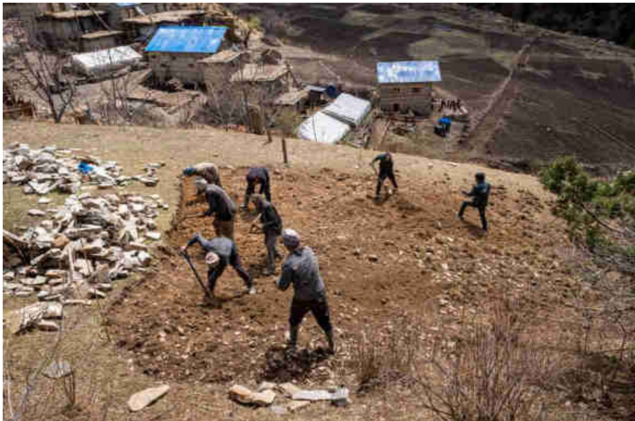
Pic. 101: Flatting the ground for the power house building structure
