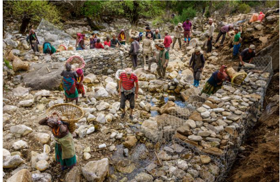
Pic. 84: Securing the sedimentation tank and water intake with gabon wires
