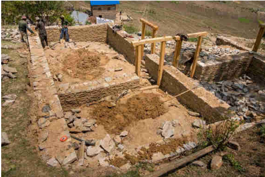
Pic. 117: Power house first floor walls building structure
