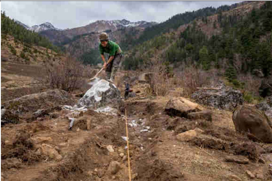
Pic 4: Clearing the HDPE penstock pipeline path from large rocks
