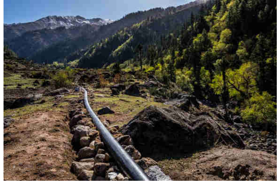
Pic. 11: Joined HDPE penstock ready for pressure test before being covered
