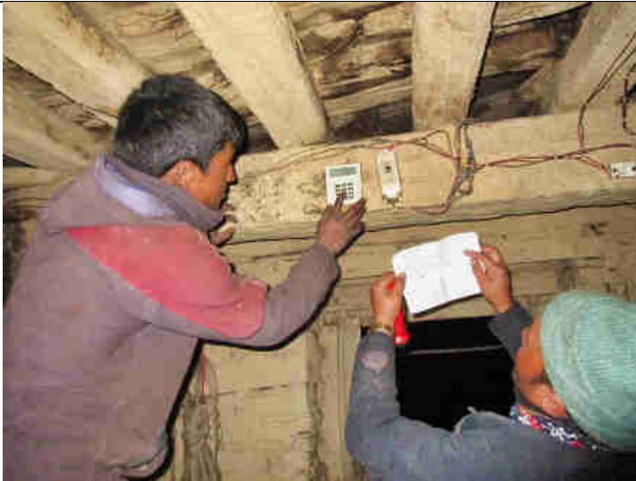
Pic 7: Operator Hiralal (left) instructs a home owner how to input the digital code for his monthly pre-paid electricity units for his home
