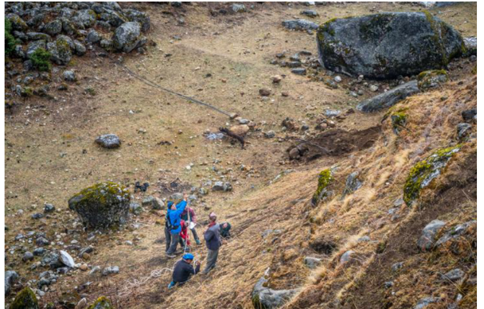
Pic. 10: The last part of the penstock has the highest drop of 20 meters
