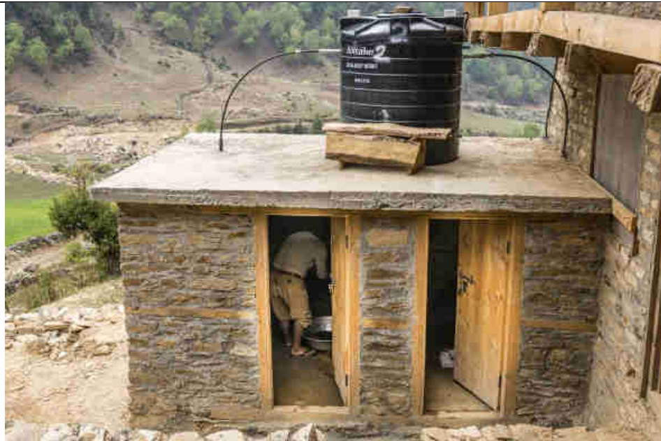
Pic 25: Power/Community house hot water shower (part of the regulated "smart" dump load, based on the power generation and the village's power demand)
