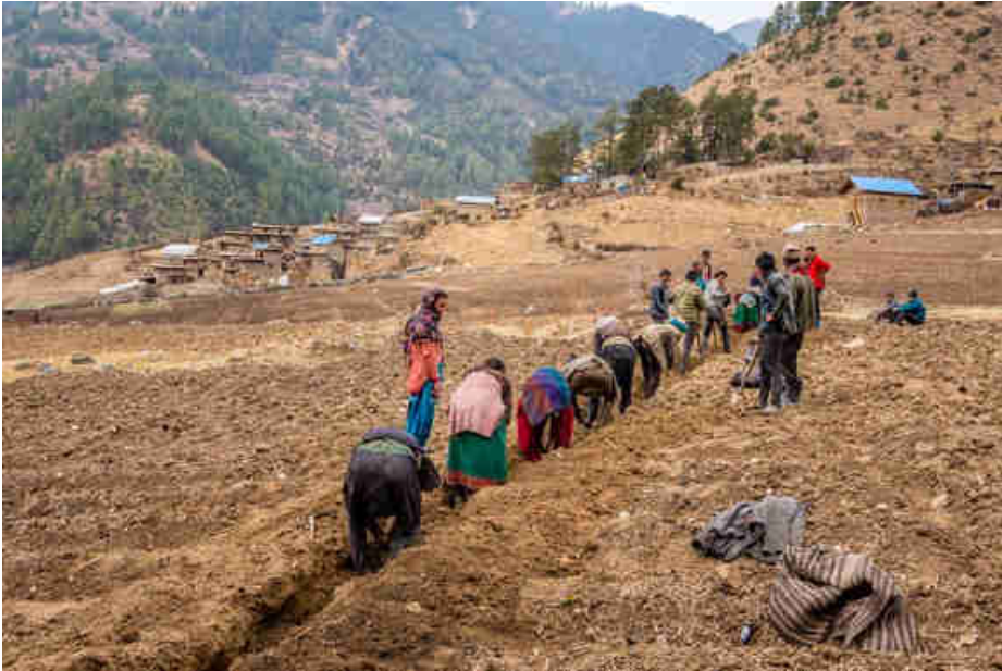
Pic. 19: Digging the canal for the underground power and communication cables
