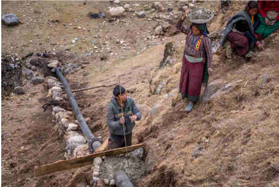
Pic. 51: The steep penstock drop is anchored and secured with cement
