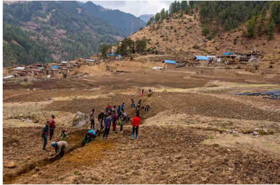
Pic. 34: Covering the power and communication cables with soil for protection
