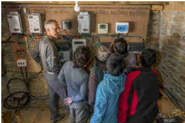
Pics. 110-112: Training of the RIDS staff and operators in the use of all the equipment in the power room by Mr. Mark Staumbaugh. In turn, the RIDS staff is training the local Mohari operators and village elders in understanding what all the pieces of equipment mean and indicate of the Modular Pico-Hydro power plant.
