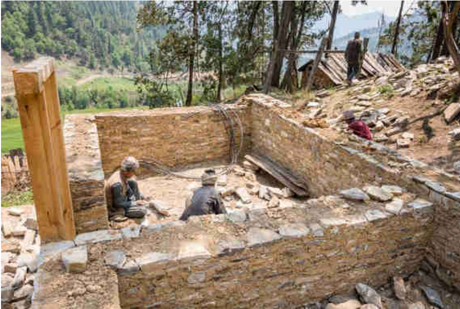
Pic. 119: Building the ground walls of the power house stone walls
