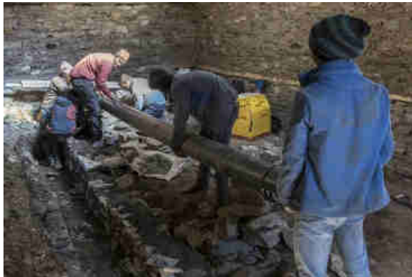
Pics. 55-57: Inside the Pico Hydro Power Plant Turbine house. The last piece (of total 92) of the 5m long HDPE PN6 200 mm diameter penstock is installed and the water canal, to install the 6 Pelton turbines, is built. The 6 PowerSpout Pelton Turbines are installed (screwed on) on top of seasoned hard wood which is resistant to water for 20 years.
