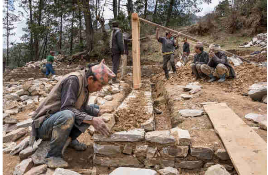
Pic. 104: Building the ground walls of the power house
