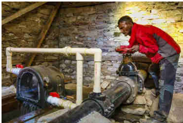
Pics. 101-103: Training of the RIDS staff how to start and stop the Modular Pico hydro-Power plant by Dr. Alex Zahnd. In turn, the RIDS staff is training the local Mohari operators and village elders in the Operation & Maintenance of the Mohari Modular Pico hydro-Power plant.
