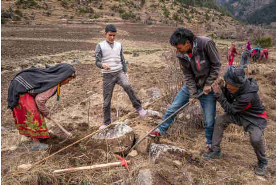
Pic. 15: Clearing the HDPE penstock pipeline path from large rocks
