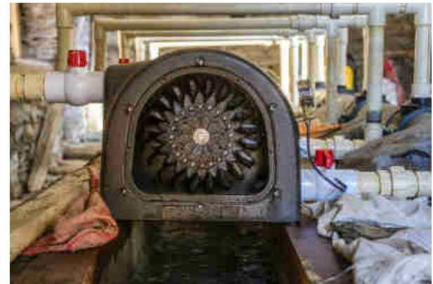
Pics 73-75. Connecting new, armoured cables to the Pelton turbines so that the cables can be put underground inside the turbine house. Each PowerSpout Pelton turbine has 48 stator fingers with a rotor with 48 permanent magnets. Each PowerSpout Pelton turbine generates at 50m head and 4 L/s water 320 Volt DC, which is sent via underground, armoured copper cables (4 x 2mm 2 size) to the 300 meter away Power House.
