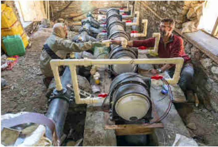
Pics. 70-72: 2" PVC piping installation to connect all the 6 Pelton turbines to the HDPE penstock.
