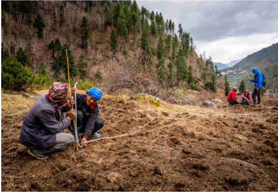
Pic. 7: The penstock pipe line is surveyed several times
