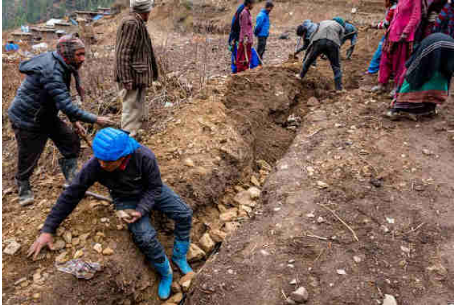
Pic. 31: Buring the cables from the turbine to the power house
