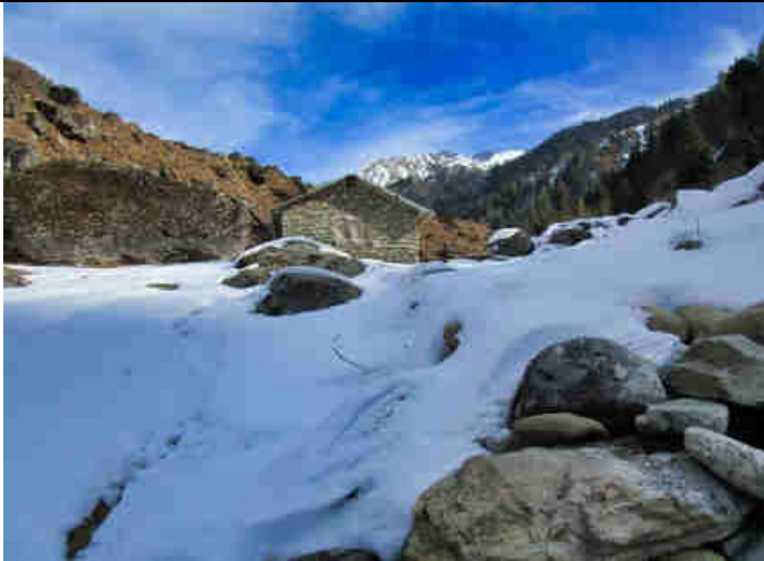
Pic 1: Mohari Modular Pico-Hydro Power Plant Turbine house with the 6 Pelton turbines during the winter 2019/2020
