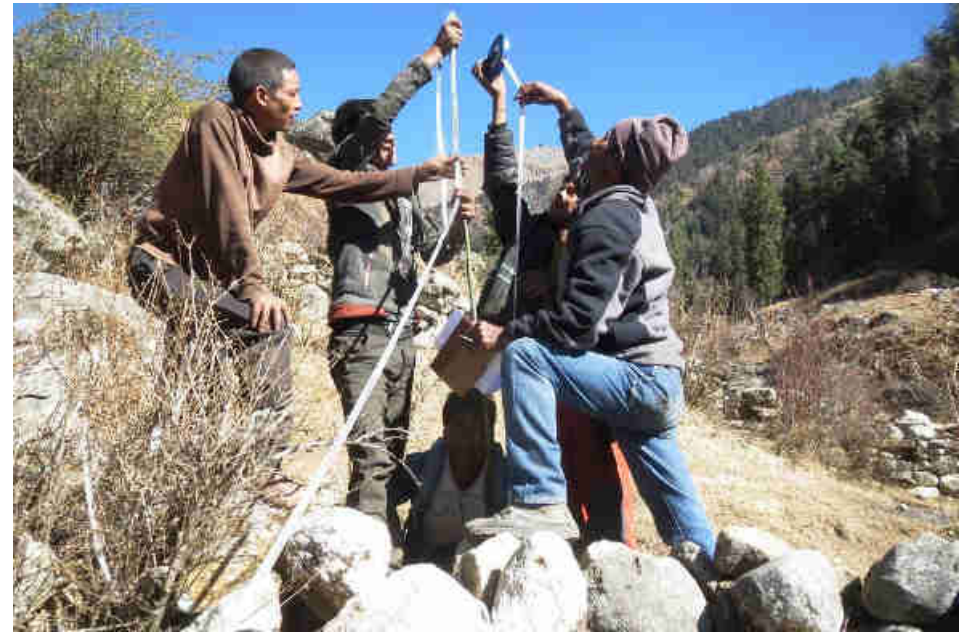
Fig. 20: Mohari village community and RIDS-Nepal Jumla staff conducting the base line survey for modular pico-hydro power plant for the Mohari village. Here they are measuring the head height from the river water intake tank to the turbine house, applying along the whole pen stock pipe the water tube method which results in the total gross head. A technology which RIDS-Nepal taught the local Mohari village user group.
