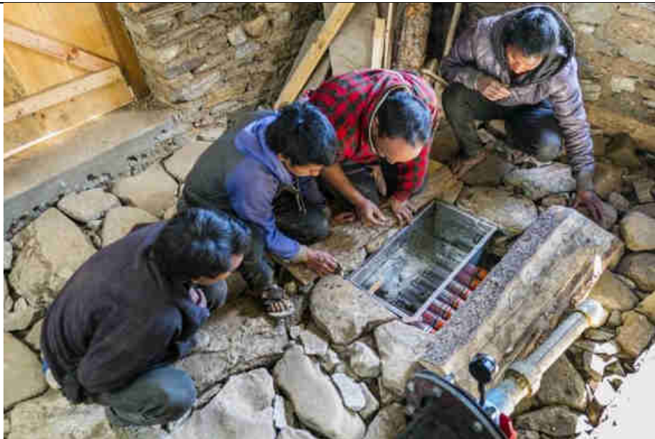
Pic. 24: Emergency, 8 kW resistor water heater in the turbine house
