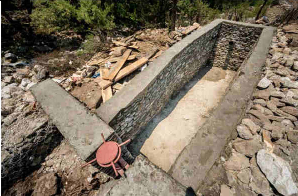
Pic. 16: Sluice gate, sedimentation tank, penstock intake, washout, overflow
