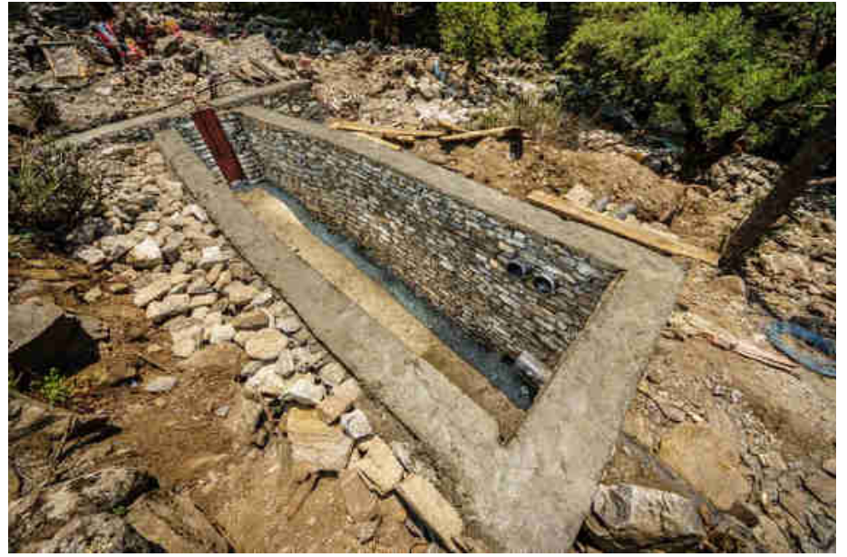
Pic. 98: Sluice gate, sedimentation tank, penstock intake, washout, overflow
