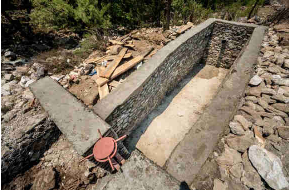
Pic. 99: Sluice gate, sedimentation tank, penstock intake, washout, overflow
