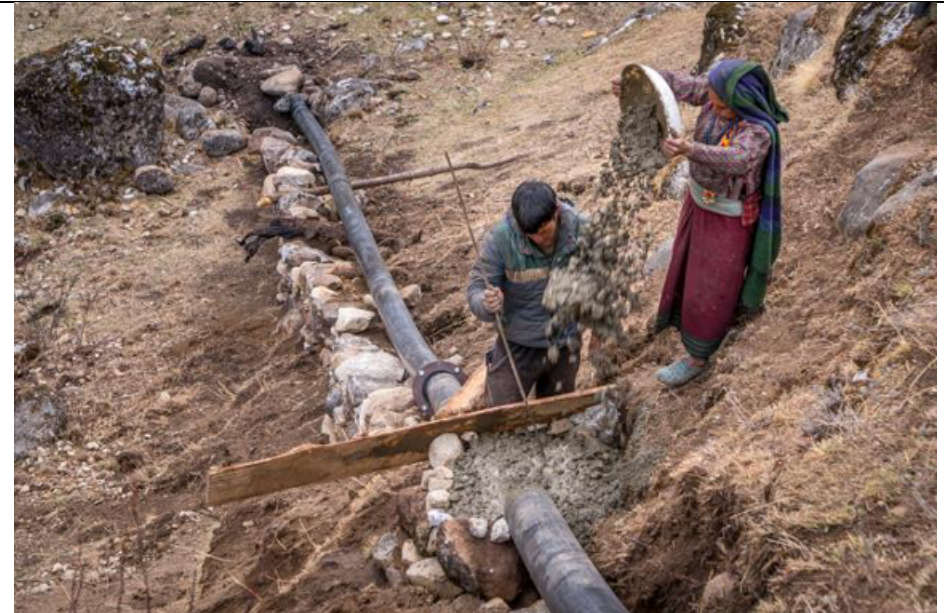
Pic. 9: The steep penstock drop is anchored and secured with cement
