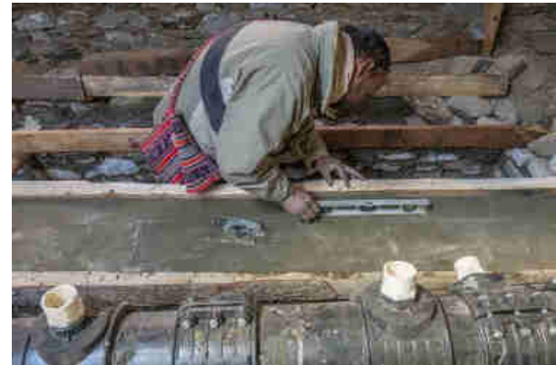
Pics. 61-63: Building the water canal for the 6 PowerSpout Pelton Turbines to be screwed on top of the seasoned hard wood. The purposely built stone wall is cemented so that it lasts for years to come and so that it is leveled for the PowerSpout Pelton Turbines.
