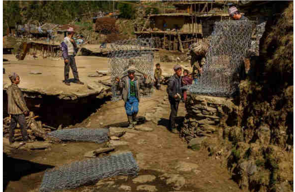
Pic. 80: Gabion wire boxes to streamline the river and secure the water intake
