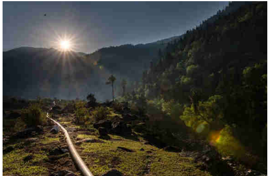
Pic. 74: Sunrise over the modular pico-hydro power penstock pipeline
