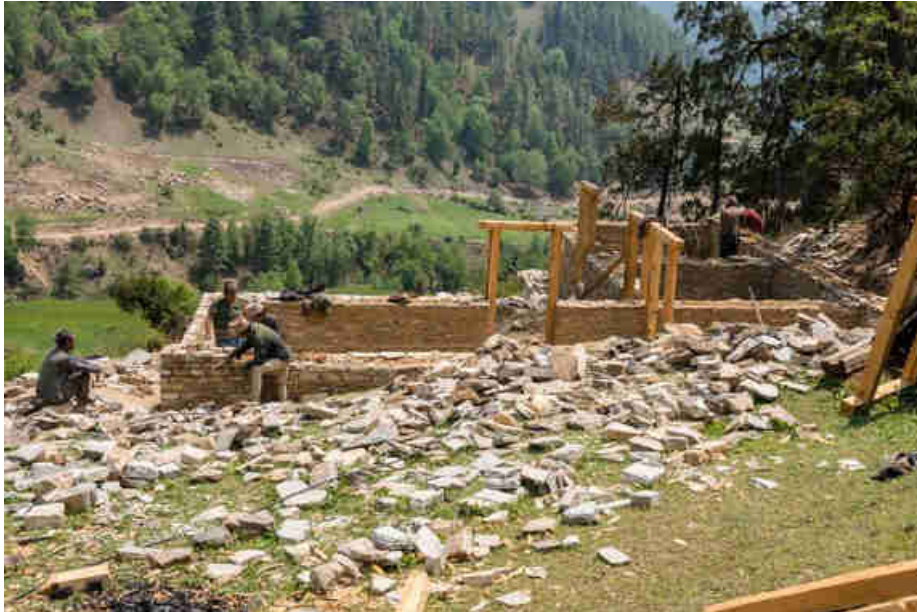
Pic. 115: Building the ground walls of the power house stone walls
