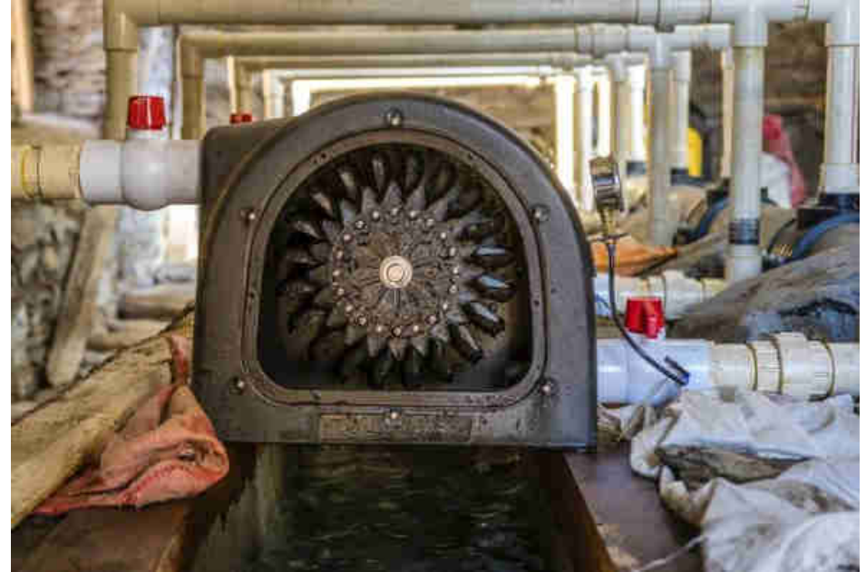
Pic. 23: PowerSpout Pelton turbine, generation 1.2kW at 40m head and 4 L/s water
