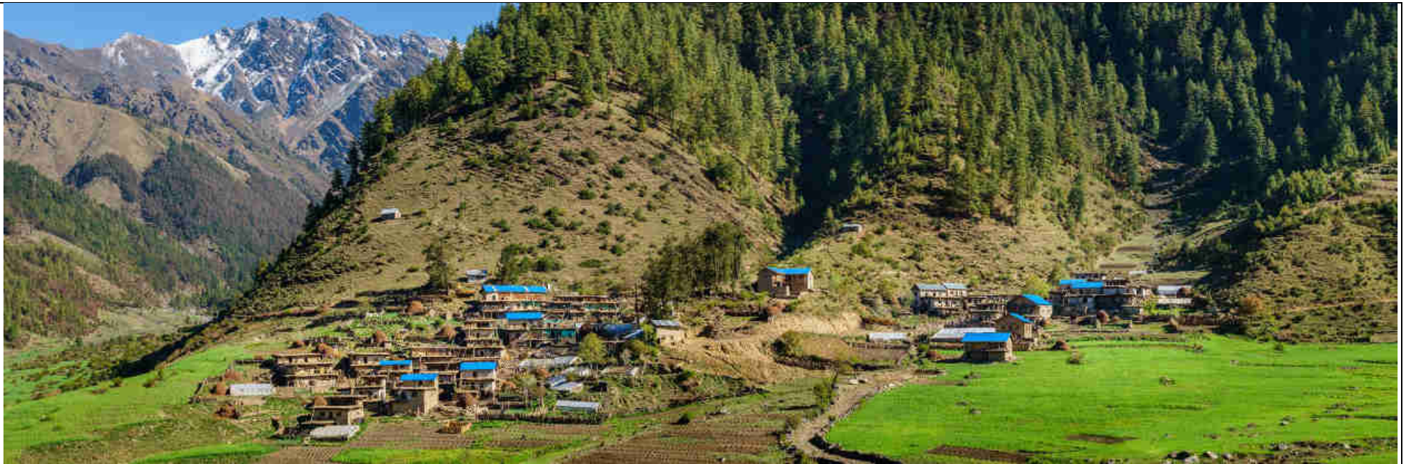
Pic 52: Mohari village fully electrified through armored underground cables into each home, saving precious Himalayan pine trees for poles. That not only increases the security for uninterrupted electricity through snow, storms, floods and rains, but actively fights the fast increasing deforestation Nepal faces nationwide.
