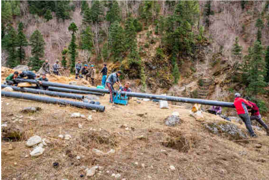
Pic. 43: Challenging environment to weld the HDPE pipes for the penstock
