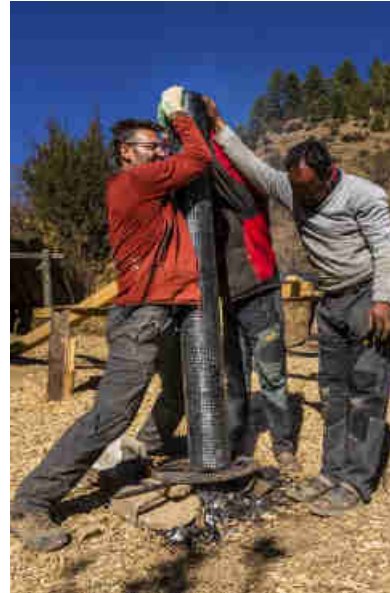
Pics. 85-87: Improving the sluice gate and HDPE intake filter, with 1060 x 8mm holes to protect the Pelton turbines from any particulates larger than 8 mm.
