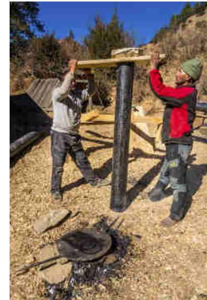
Pics. 85-87: Improving the sluice gate and HDPE intake filter, with 1060 x 8mm holes to protect the Pelton turbines from any particulates larger than 8 mm.
