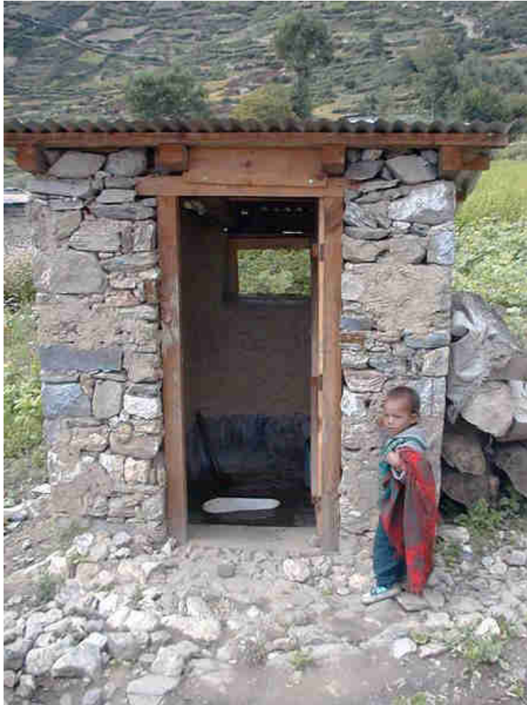
Fig 3: Pit Latrine in Mohari Village, one per family
