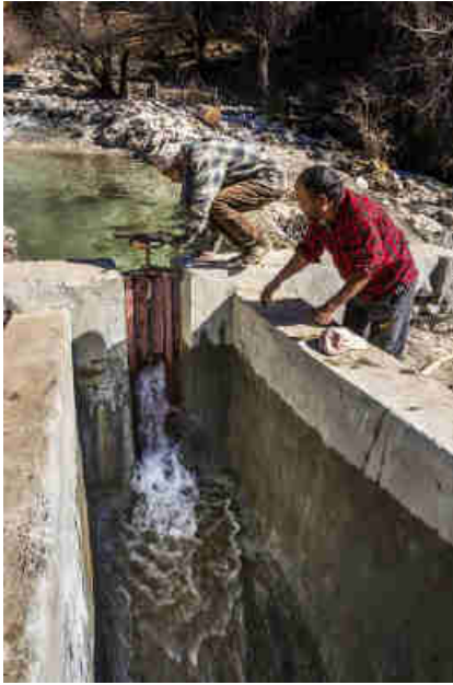
Pics. 82-84: RIDS staff training the two local operators, Aitaram and Hiralal, how to operate and maintain the sluice gate valve of the sedimentation tank.
