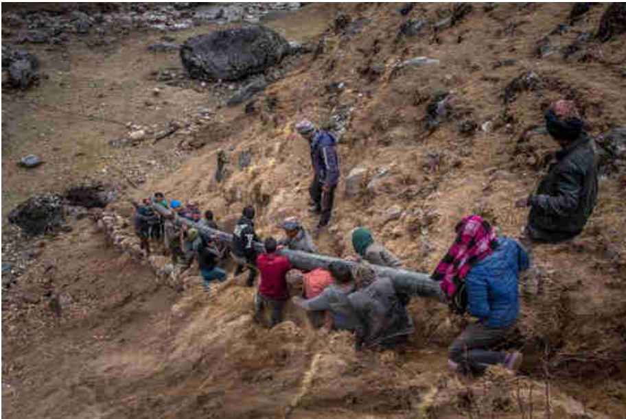
Pic. 65: Bringing the steep sloped HDPE penstock pipe into place
