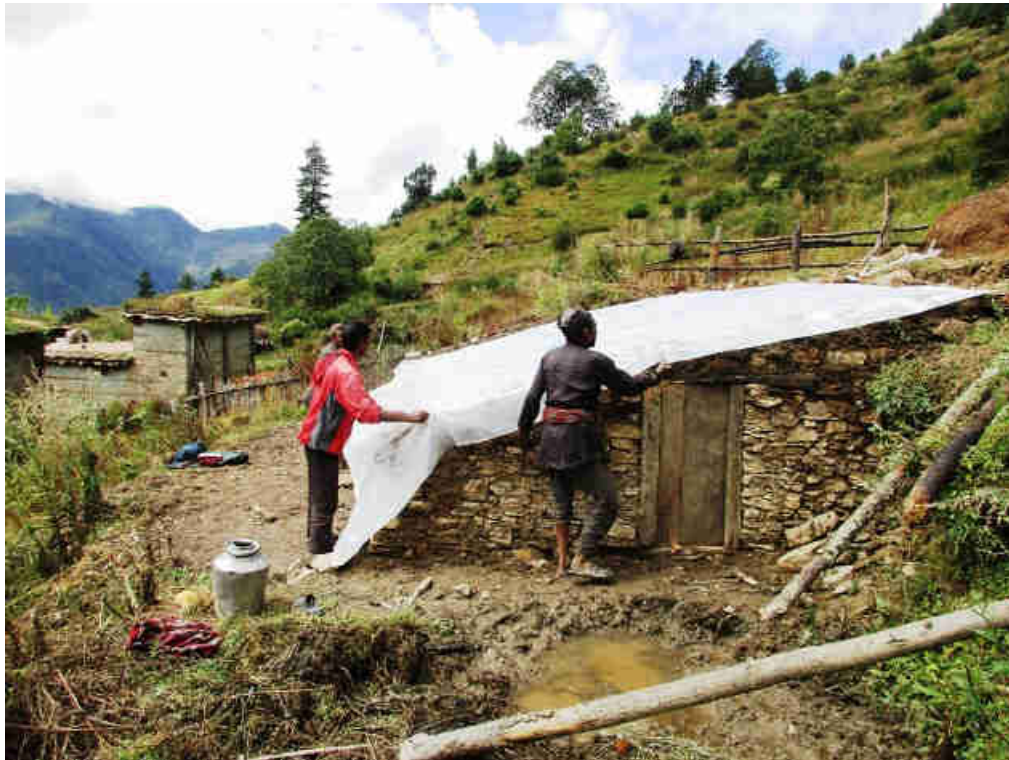
Fig. 11: RIDS-Nepal staff instruct and teach the local farmers and families from Mohari village how a high-altitude greenhouse is built, crops are planted and cared for throughout the year.
