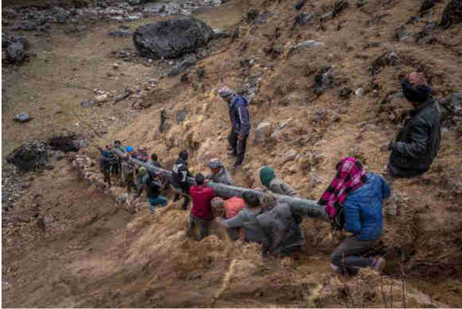
Pic. 10: Bringing the steep sloped HDPE penstock pipe into place
