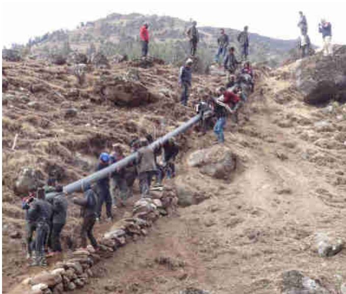
Fig. 15: Laying Penstock in Steep Section
