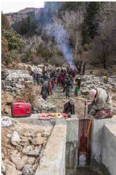
Pics. 85-87: Improving the sluice gate and HDPE intake filter, with 1060 x 8mm holes to protect the Pelton turbines from any particulates larger than 8 mm.
