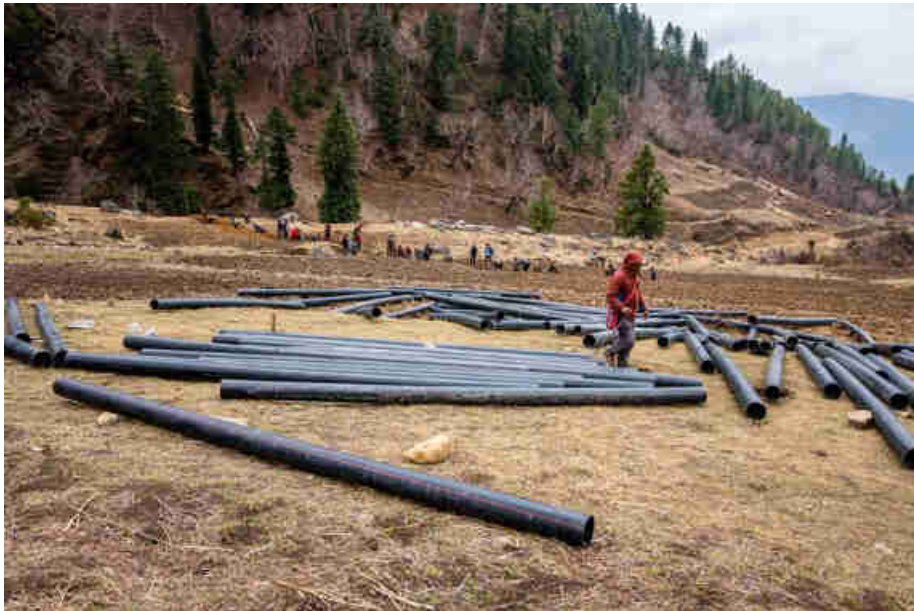
Pic. 25: The various HDPE penstock pipes based on the pressure/head
