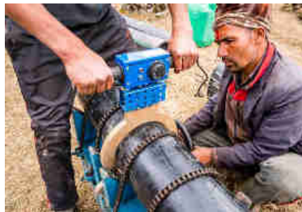
Fig. 3: Thermally Welding the Penstock
