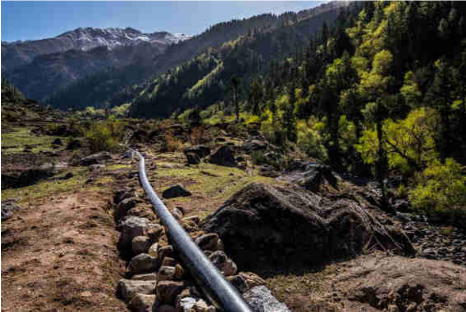
Pic. 63: Joined HDPE penstock ready for pressure test before being covered
