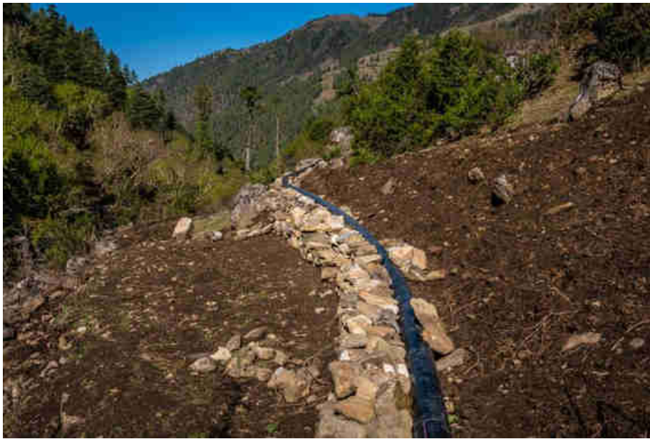
Pic. 53: Welded 200mm diameter HDPE penstock ready for the pressure test
