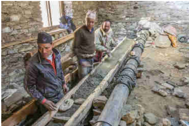
Pics. 61-63: Building the water canal for the 6 PowerSpout Pelton Turbines to be screwed on top of the seasoned hard wood. The purposely built stone wall is cemented so that it lasts for years to come and so that it is leveled for the PowerSpout Pelton Turbines.
