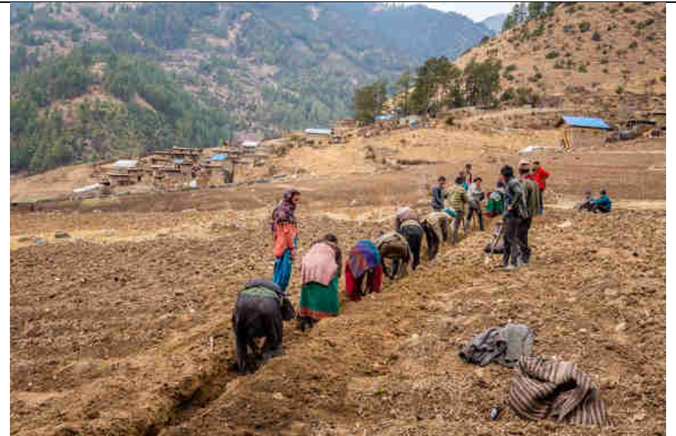
Pic 5: Digging the canal for the underground power and communication cables
