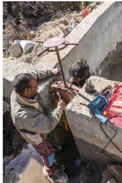
Pics. 85-87: Improving the sluice gate and HDPE intake filter, with 1060 x 8mm holes to protect the Pelton turbines from any particulates larger than 8 mm.
