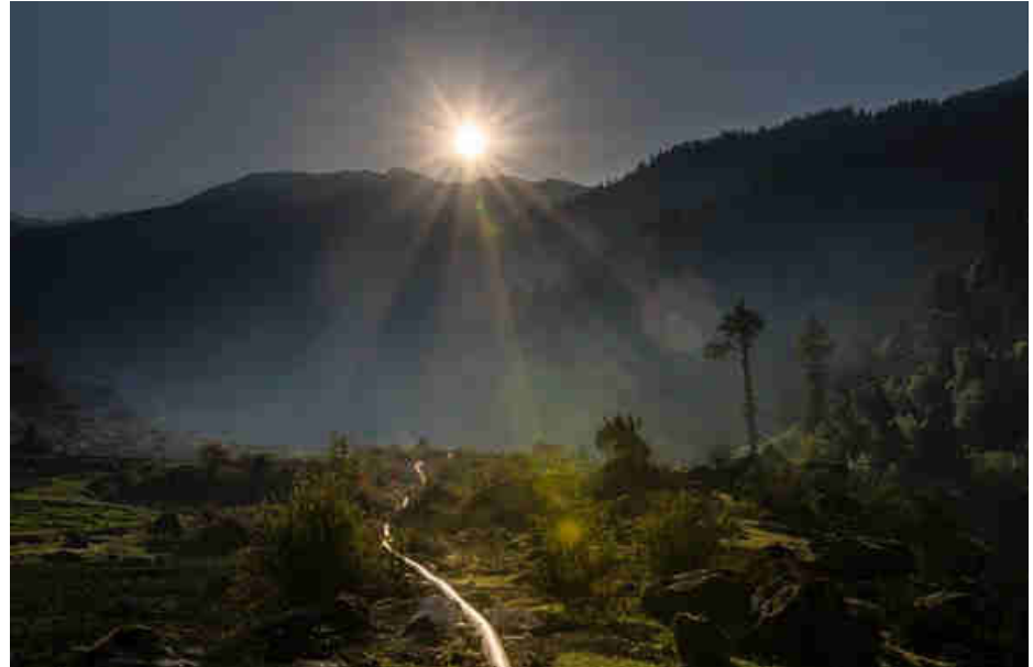
Pic. 76: The sun over the modular pico-hydro power penstock pipeline
