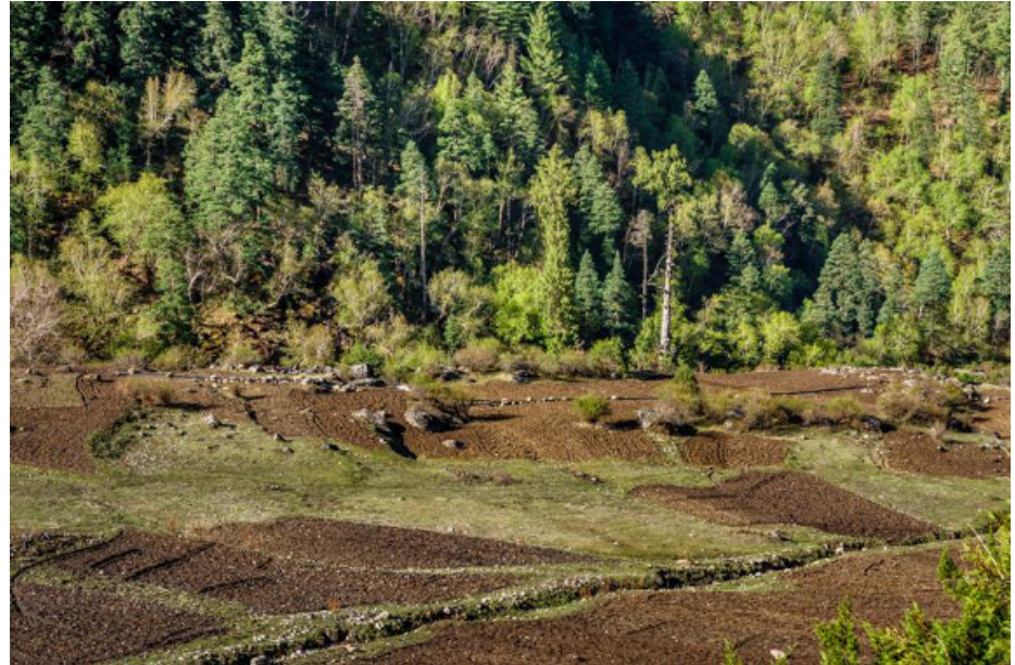
Pic. 60: The 455 m long HDPE penstock pipe line through fields
