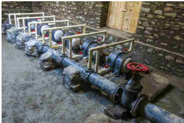
Pics. 134-136: Left: Modular Pico-Hydro Power on the 30 th Nov. 2018. Middle: 5.61 kW Power generation. Aim was to achieve 5 kW, so aim fulfilled! Right: First movie and slide evening with over 120 local people taking part and enjoying the first community hall evening in the power/community house.
