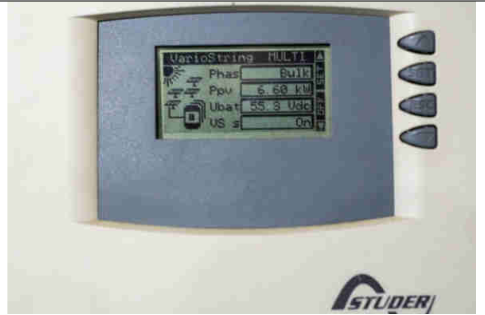
Pic. 31: 6.6 kW Power generation with 6 turbines at 47 m head and 20 L/sec = 72%
