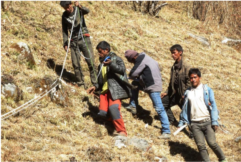
Fig. 19: Mohari village community and RIDS-Nepal Jumla staff conducting the survey for the modular pico-hydro power plant for the Mohari village. Here the people are measuring the length of the pen stock pipe, which will be buried underground, from the water intake tank to the turbine house. The person to the very right is the RIDS-Nepal sponsored Karnali Technical School sub-overseer student who puts to work some of his newly learned knowledge. He will be a potential future pico-hydro power plant operator once he finished his studies and the Mohari modular pic-hydro power plant is built and running.
