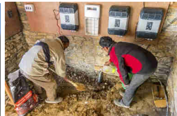
Pics 98-100: Building the Super-Earthing system in the Turbine house (left) and the Power Room in the Power/Community House in the village (right) to make sure the whole Modular Pico-Hydr Power Plant is protected with a correct and proper earthing system.
