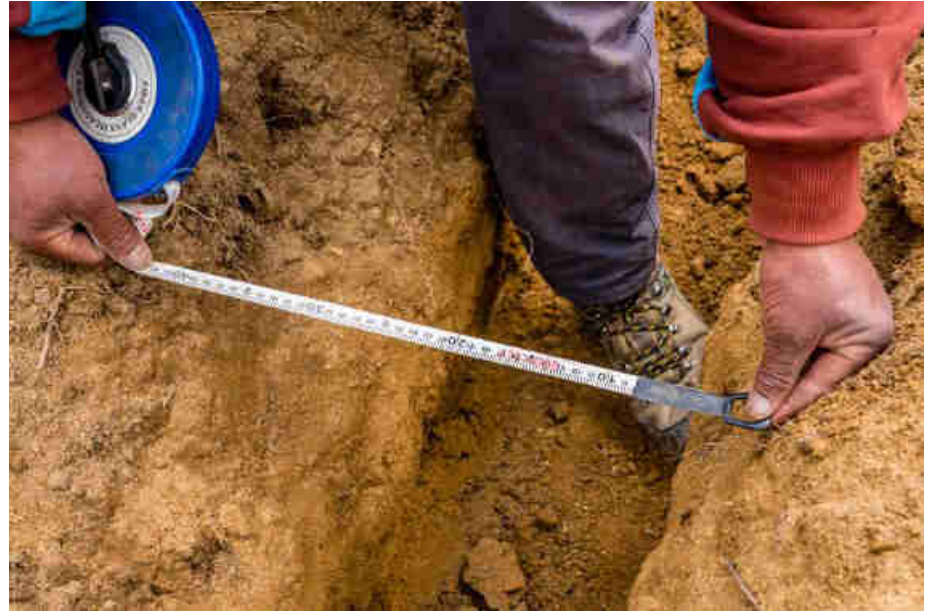
Pic. 24: Digging the 400cm wide canal for the underground cables
