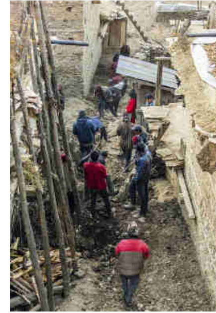
Pics. 27-29: All main and house cabling is through armoured, underground cables, so the Mohari families had to dig trenches for all cables to reach the homes.
