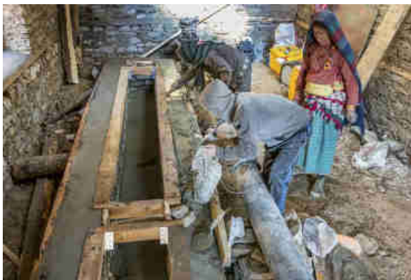
Pics. 61-63: Building the water canal for the 6 PowerSpout Pelton Turbines to be screwed on top of the seasoned hard wood. The purposely built stone wall is cemented so that it lasts for years to come and so that it is leveled for the PowerSpout Pelton Turbines.
