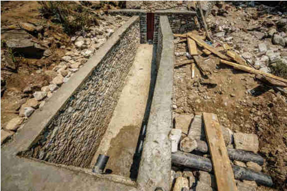
Pic. 97: :Sluice gate, sedimentation tank, penstock intake, overflow
