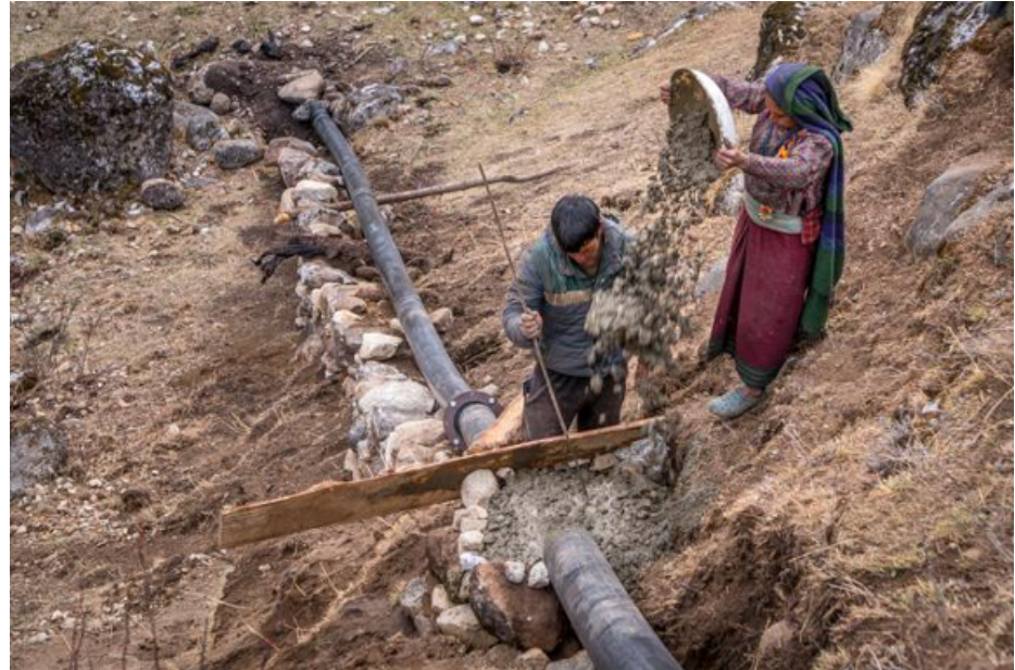
Pic. 52: The steep penstock drop is anchored and secured with cement
