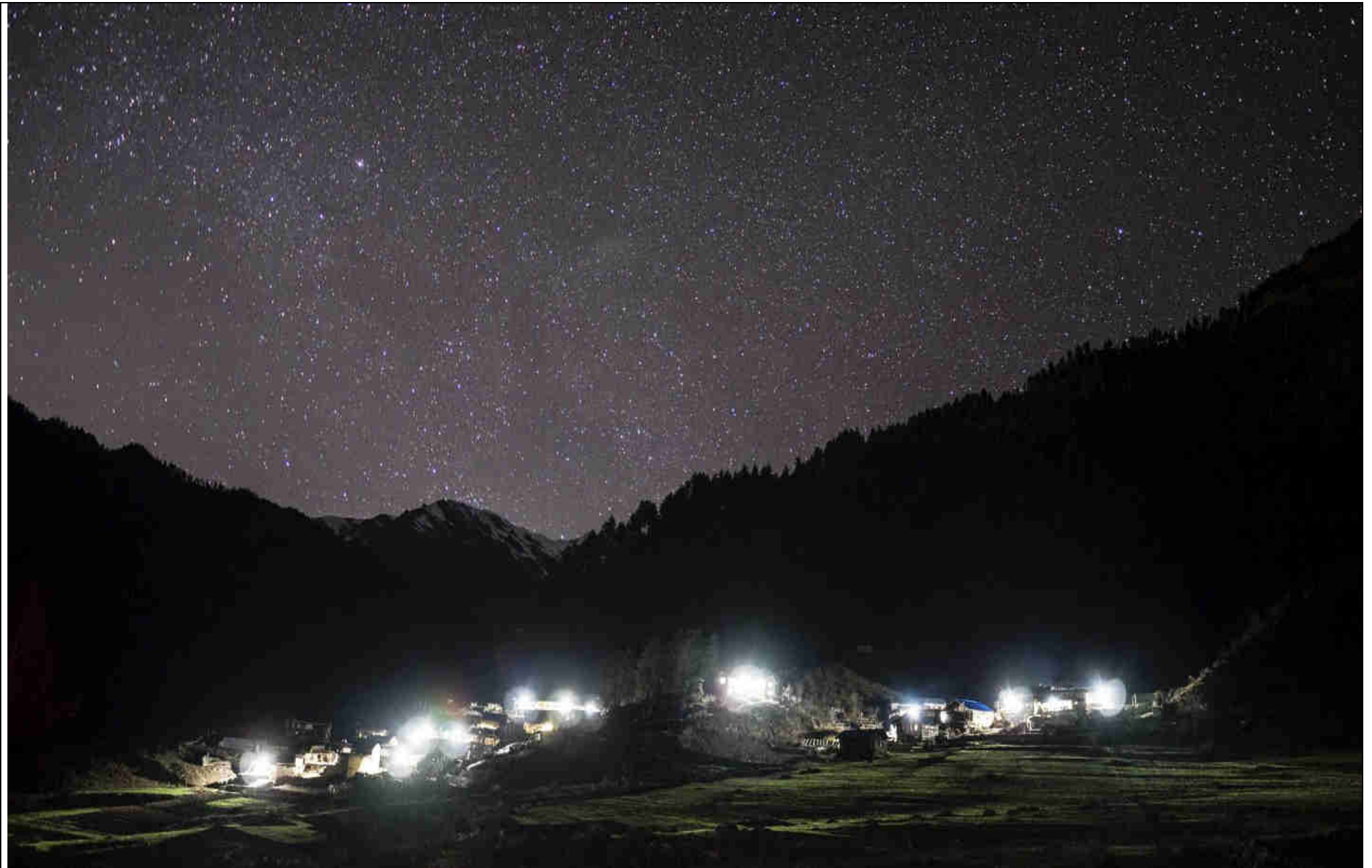
Pic 47: Mohari Village by night with the Modular Pico-Hydro Power Plant generating electricity for all demanded energy services of the village and power/community center
