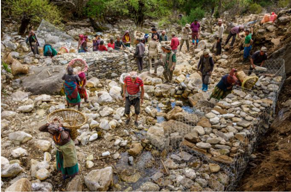
Pic. 14: Securing the sedimentation tank and water intake with gabion wires
