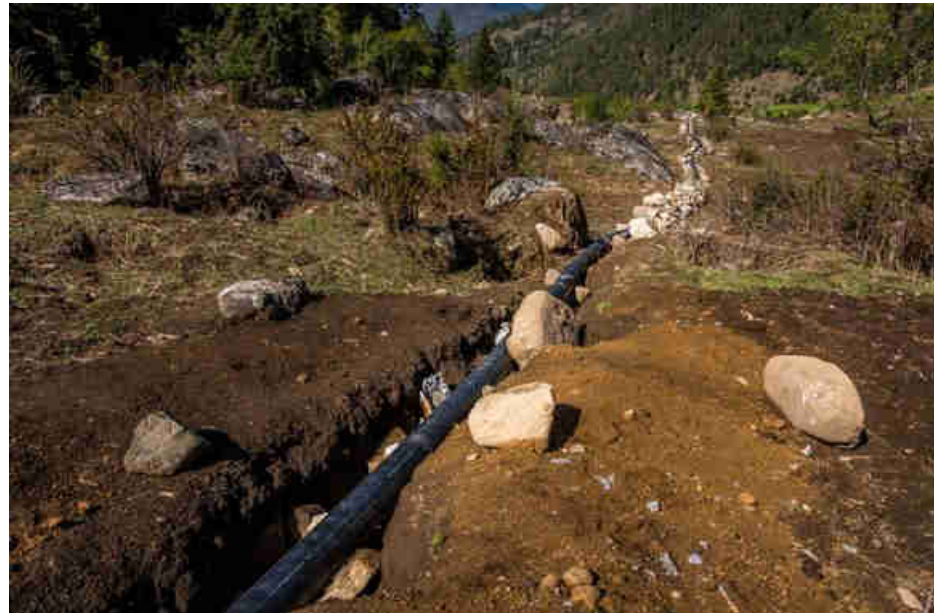
Pic. 62: Joined HDPE penstock ready for pressure test before being covered
