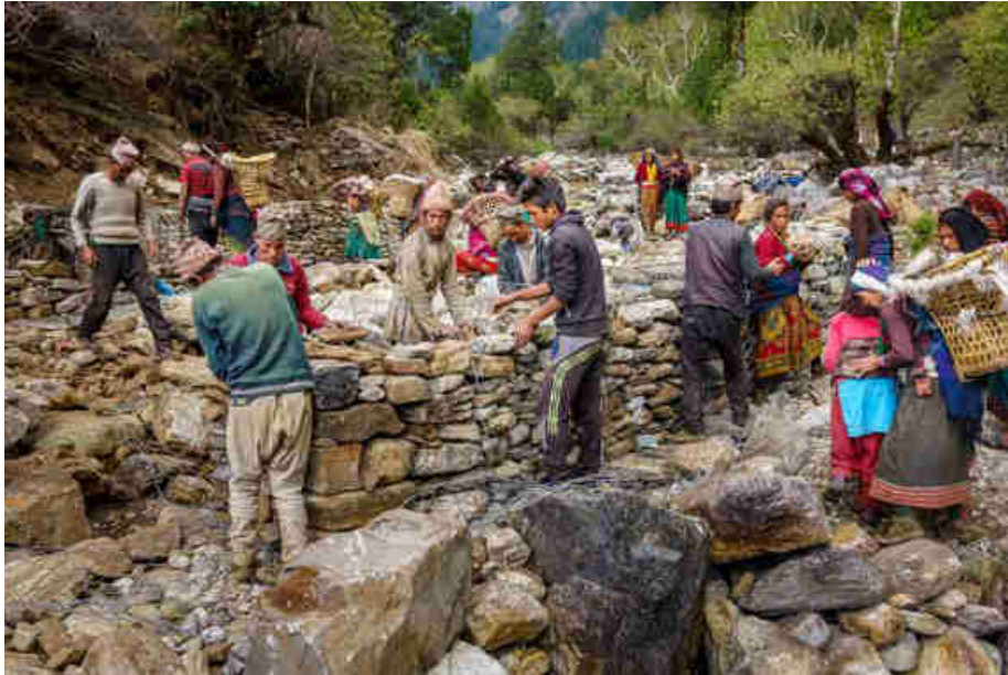
Pic. 83: Securing the sedimentation tank and water intake with gabon wires
