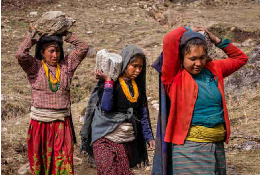
Pic. 87: Women carrying stones for the gabon wire protection boxes
