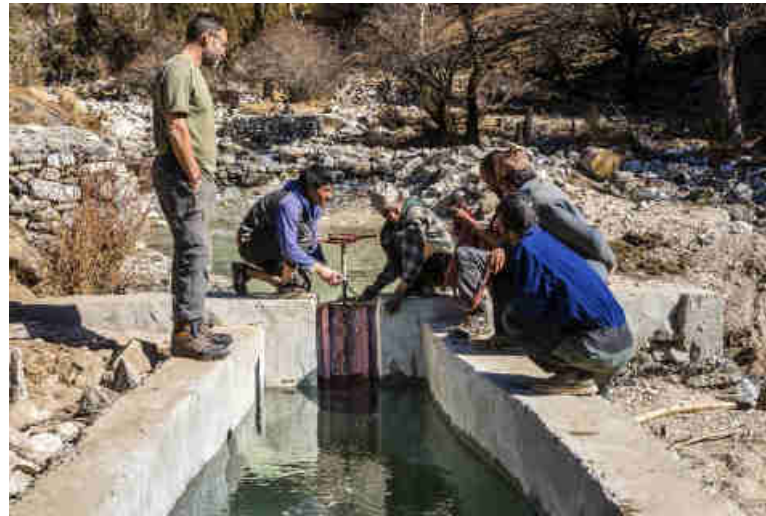
Pics. 82-84: RIDS staff training the two local operators, Aitaram and Hiralal, how to operate and maintain the sluice gate valve of the sedimentation tank.
