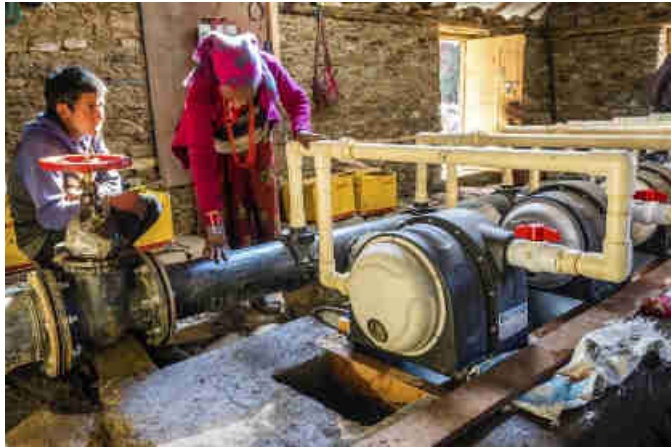
Pics. 107-109: Training of the local Mohari operator Hiralal Buddha with a local woman checking out the new pico power plant. The electronic system in turbine house (right) to assure that the needed DC voltage is achieved and maintained during the operation of the 6 turbines.
