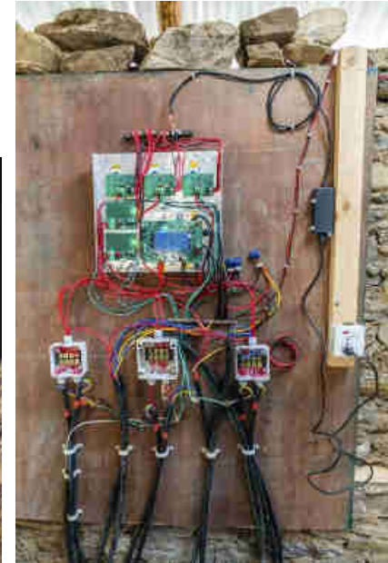
Pics. 107-109: Training of the local Mohari operator Hiralal Buddha with a local woman checking out the new pico power plant. The electronic system in turbine house (right) to assure that the needed DC voltage is achieved and maintained during the operation of the 6 turbines.
