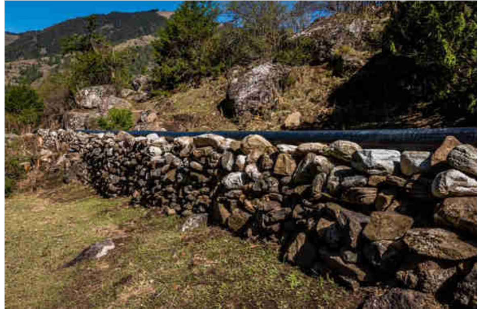
Pic. 64: Joined HDPE penstock ready for pressure test before being covered
