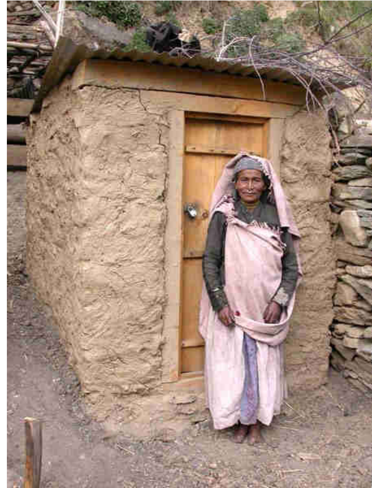
Fig 4: Pit Latrine in Mohari Village, which each family built under RIDS' instructions
