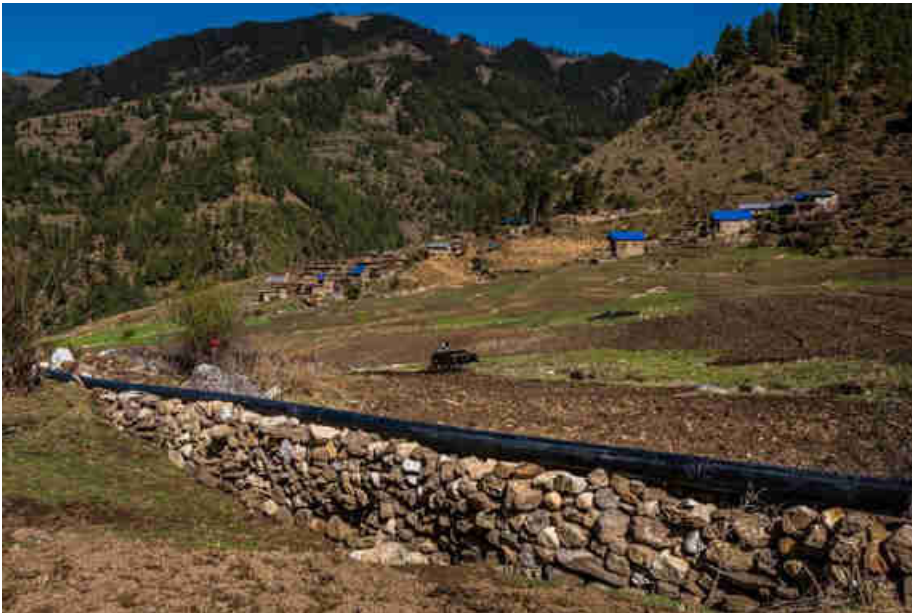
Pic. 61: Joined HDPE penstock pipes before being buried
