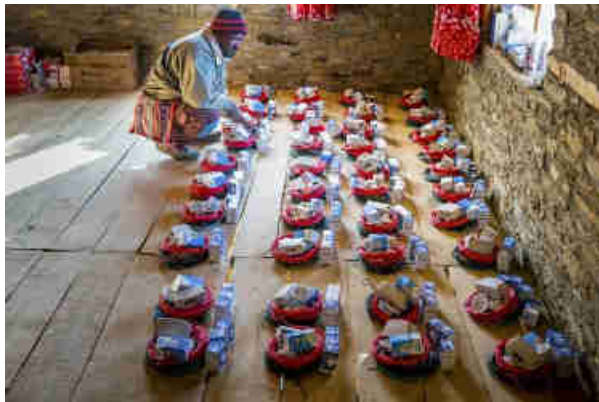
Pics. 43-45: House wiring equipment for each of the 42 homes in Mohari village. 20 m red and black cables, 4 LED lights (3 x 3watt and 1 x 5 watt), 4 bulb connectors and switches, PAYG meter, 2 Ampere MCB and insulation tape, is made available for each household to be picked up before the installation.
