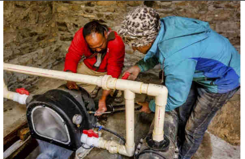
Pic. 35: Monthly greasing of each turbine while continuing generating electricity
