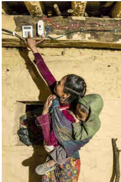
Pics. 122-124: Pre-payment display and 2 Amps MCB (left) and light inside 3-4 rooms in each of the Mohari family home.
