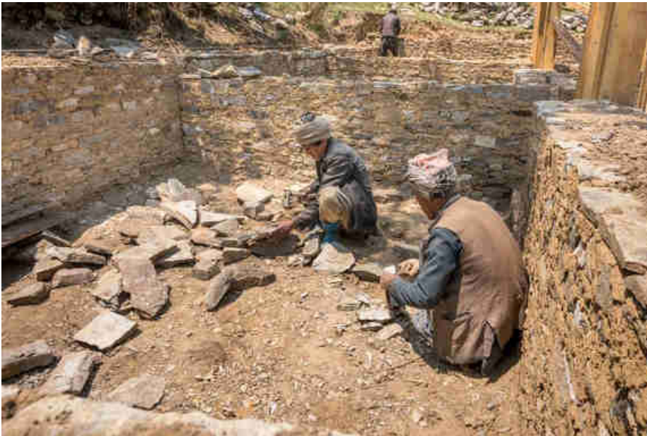
Pic. 121: Stone masonry work for building the stone walls
