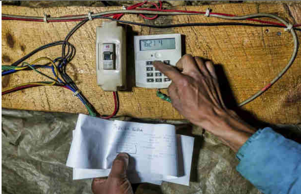
Pic 35: The unique printed token number for their paid monthly energy is input in the user's home display, connected to the dedicated smart meter to add energy units
