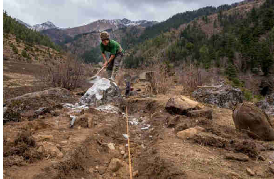
Pic. 12: Clearing the HDPE penstock pipeline path from large rocks
