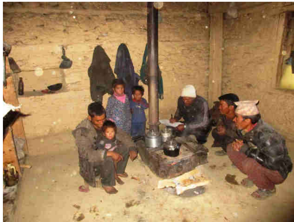
Fig 6: Smokeless Metal Stove in one of the Mohari village’s families installed. The first, RIDS-Nepal developed, smokeless metal stoves have been installed in Mohari village in 2002 and all of them are still functional and in daily use.
