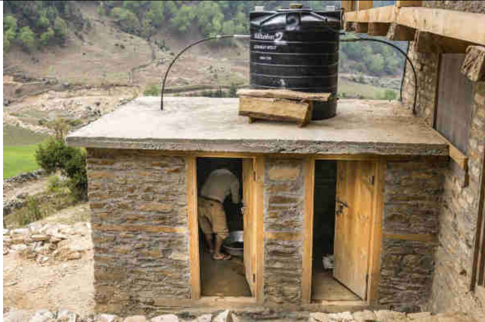
Pic. 36: Hot water shower, one of the several “smart dump” loads in the system
