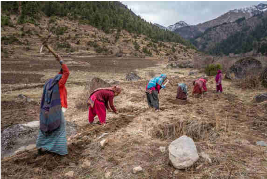
Pic. 21: Digging the path for the 200 mm diameter HDPE penstock pipes
