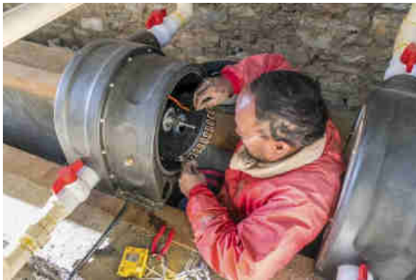
Pics 73-75. Connecting new, armoured cables to the Pelton turbines so that the cables can be put underground inside the turbine house. Each PowerSpout Pelton turbine has 48 stator fingers with a rotor with 48 permanent magnets. Each PowerSpout Pelton turbine generates at 50m head and 4 L/s water 320 Volt DC, which is sent via underground, armoured copper cables (4 x 2mm 2 size) to the 300 meter away Power House.
