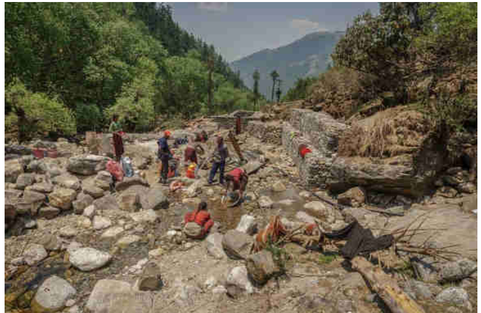
Pic. 82: Women washing the sand from mud to cement the sedimentation tank
