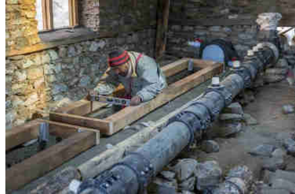
Pics. 55-57: Inside the Pico Hydro Power Plant Turbine house. The last piece (of total 92) of the 5m long HDPE PN6 200 mm diameter penstock is installed and the water canal, to install the 6 Pelton turbines, is built. The 6 PowerSpout Pelton Turbines are installed (screwed on) on top of seasoned hard wood which is resistant to water for 20 years.
