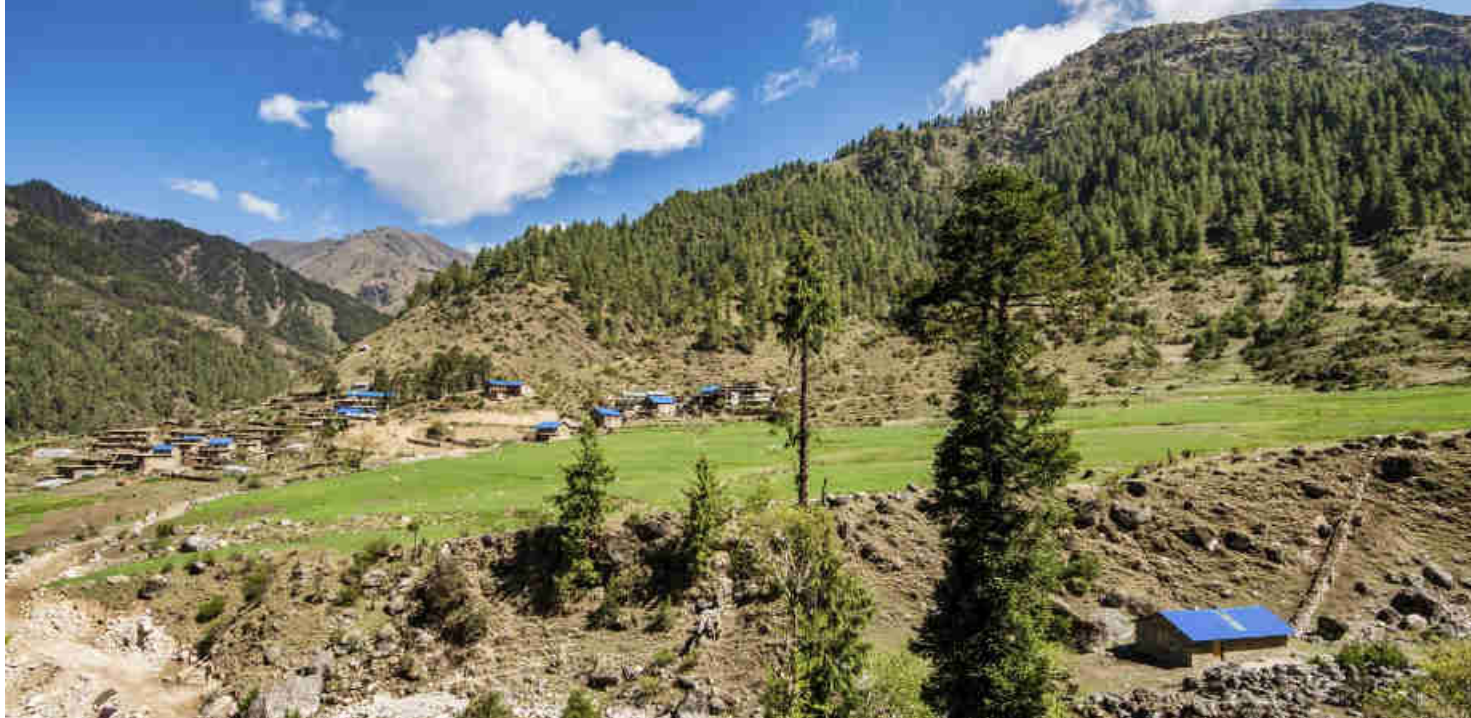
Pic 5: The modular pico-hydro power plant's turbine house with the 6 Pelton turbines is located at the bottom right, connected via armored underground cables to the 300 meters away located village and power/community house where the generated power is managed and distributed to the village and the various smart dump loads.
