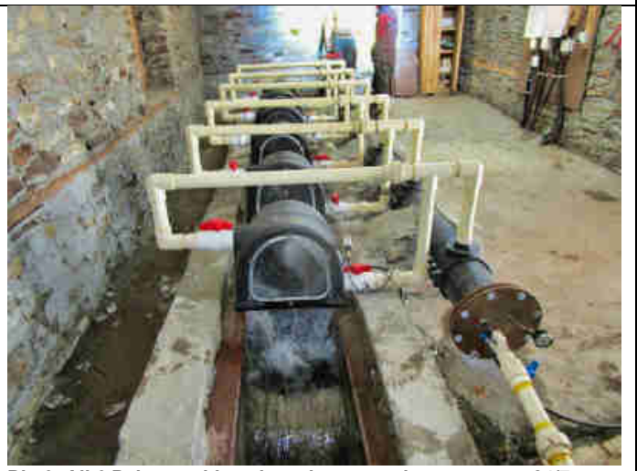
Pic 6: All 6 Pelton turbines have been running non-stop, 24/7 since the 30 th November 2018. That means that by around the 22 nd January 2020 the Mohari village Modular Pico-Hydro power plant has been running for 10'000 hours. Thus, a first milestone towards sustainability has been reached
