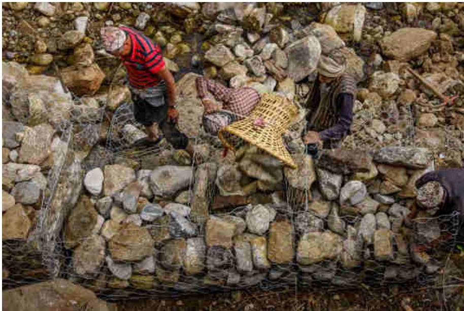
Pic. 85: Building gabon wire protection to secure the sedimentation tank
