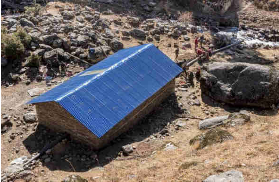
Pic. 18: Mohari pico-hydro power plant turbine house with penstock and outflow pipes
