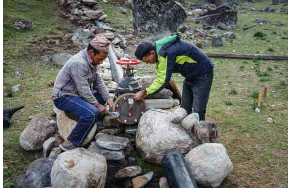
Pic. 68: Successful pressure test of each of the 91 HDPE penstock pipes
