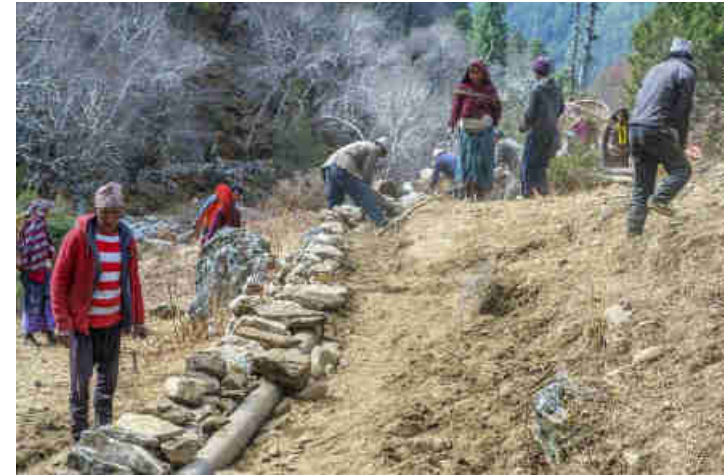
Pics. 15-17: Covering the 460 m long HDPE 200mm diameter penstock with stones and mud for increased protection from the elements and farming activities.
