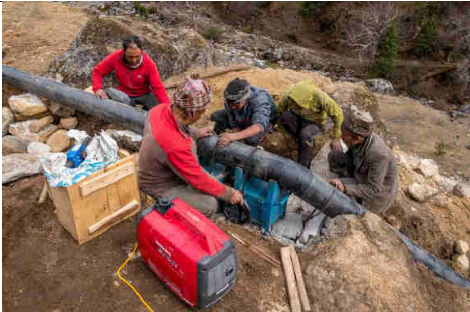
Pic. 8: Welding on the 45° elbow HDPE has been particualr a challenge
