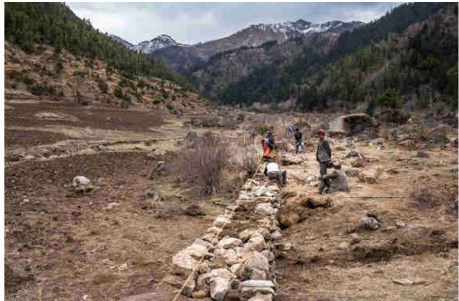
Pic. 14: Building the HDPE penstock pipeline with stone bridges etc.
