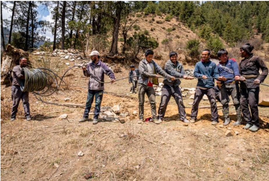
Pic. 29: Unrolling the HDPE pipe for the communication cable
