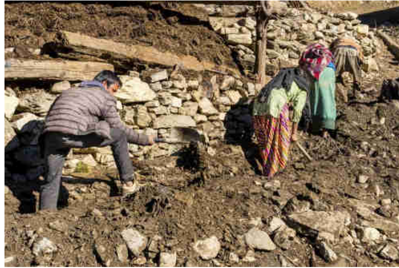
Pics. 27-29: All main and house cabling is through armoured, underground cables, so the Mohari families had to dig trenches for all cables to reach the homes.
