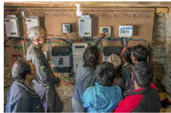
Pics. 95-97: Building the wooden box for the 200Ah 48 VDC battery bank for the Power room. Inside the power room, installing the various power electronic equipments such as the inverters, charge controllers, computer, switches and security systems.
