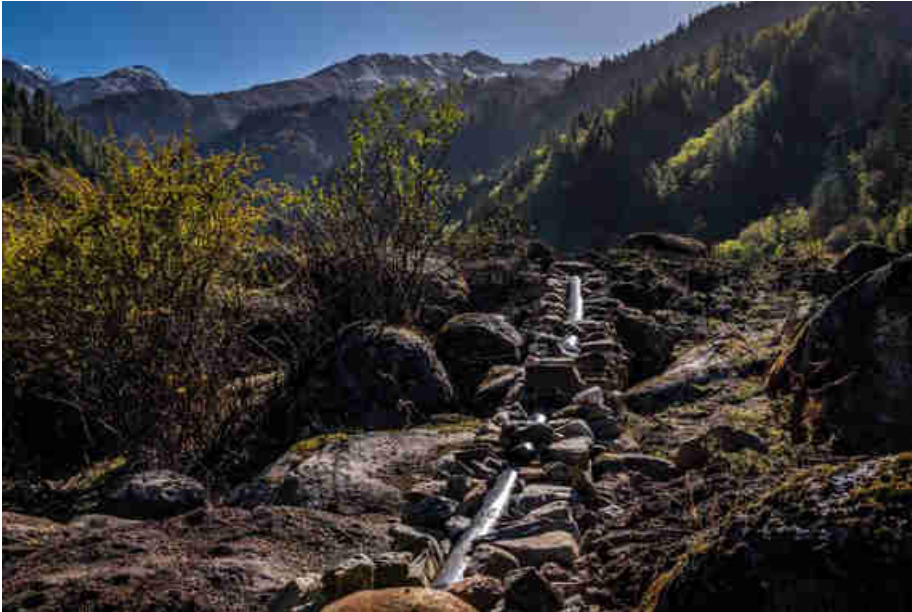
Pic. 59: Joined HDPE penstock pipes before being buried
