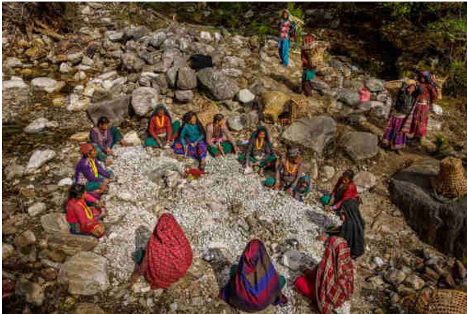
Pic. 89: Women crushing stones with a hammer for gravel for the cement
