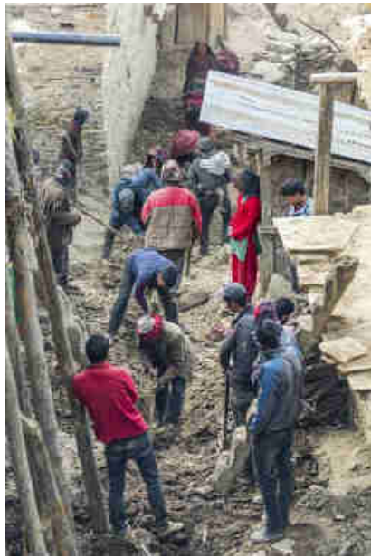
Pics. 27-29: All main and house cabling is through armoured, underground cables, so the Mohari families had to dig trenches for all cables to reach the homes.
