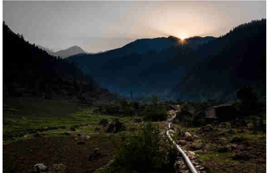
Pic. 72: Sunrise above the modular pico-hydro power penstock pipeline
