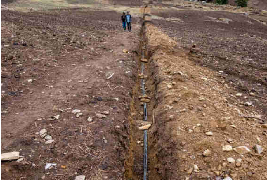
Pic. 6: Layed copper power cable and communication cable before burying them
