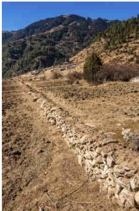
Pics. 18-20: Covered, protected 460 m long, 50 m head, HDPE penstock pipe which carries 24 liter water per second to power the 6 PowerSpout Pelton Turbines.
