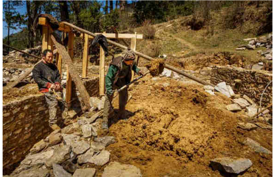
Pic. 108: Preparing the mud with water to be used as the “local cement”
