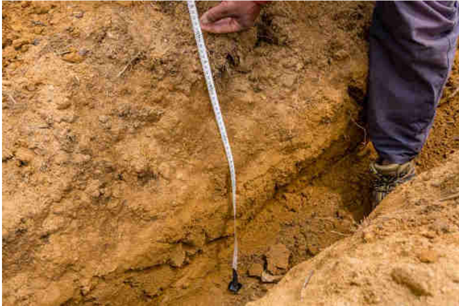
Pic. 23: Digging the 60cm deep canal for the underground cables
