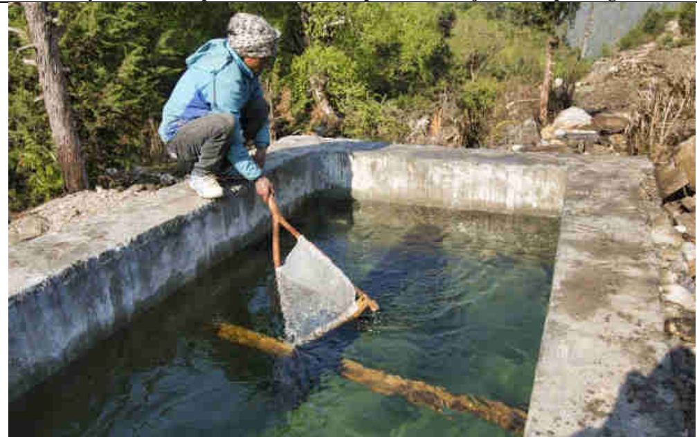
Pic 22: Daily cleaning of the HDPE intake filter at the sedimentation tank
