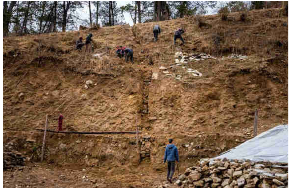
Pic. 18: Buriing the underground armoured copper cable to the power house
