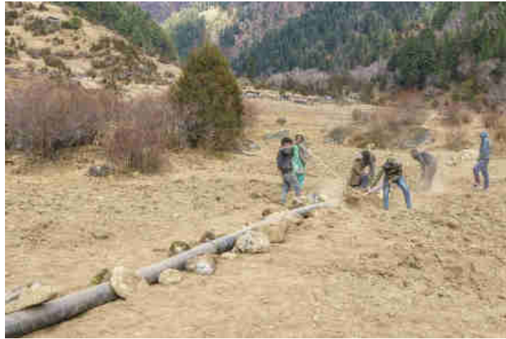
Pics. 15-17: Covering the 460 m long HDPE 200mm diameter penstock with stones and mud for increased protection from the elements and farming activities.
