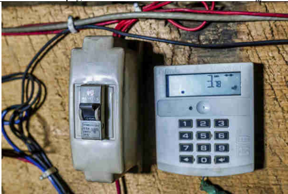
Pic 37: The smart meter registers all energy use and displays the energy left
