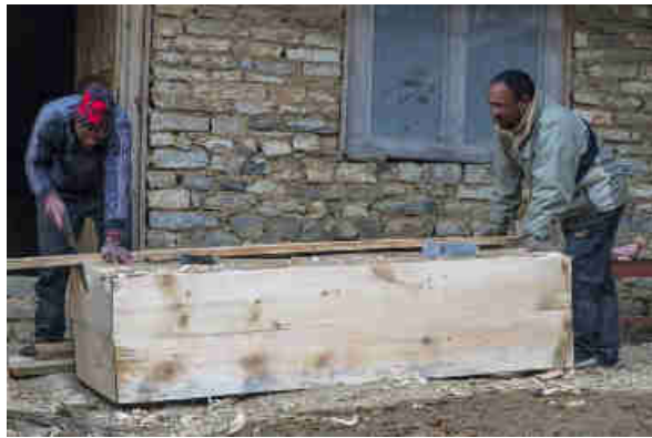
Pics. 95-97: Building the wooden box for the 200Ah 48 VDC battery bank for the Power room. Inside the power room, installing the various power electronic equipments such as the inverters, charge controllers, computer, switches and security systems.
