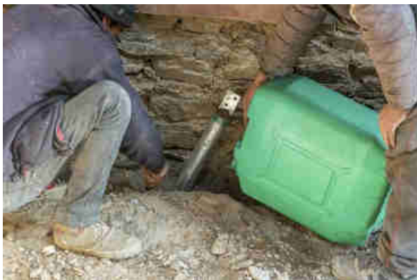
Pics 98-100: Building the Super-Earthing system in the Turbine house (left) and the Power Room in the Power/Community House in the village (right) to make sure the whole Modular Pico-Hydr Power Plant is protected with a correct and proper earthing system.
