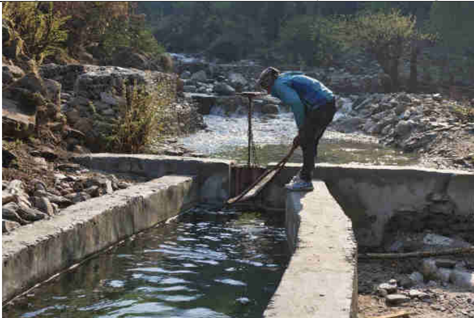
Pic 21: Daily cleaning of the sedimentation tank at the sluice gate and intake tank
