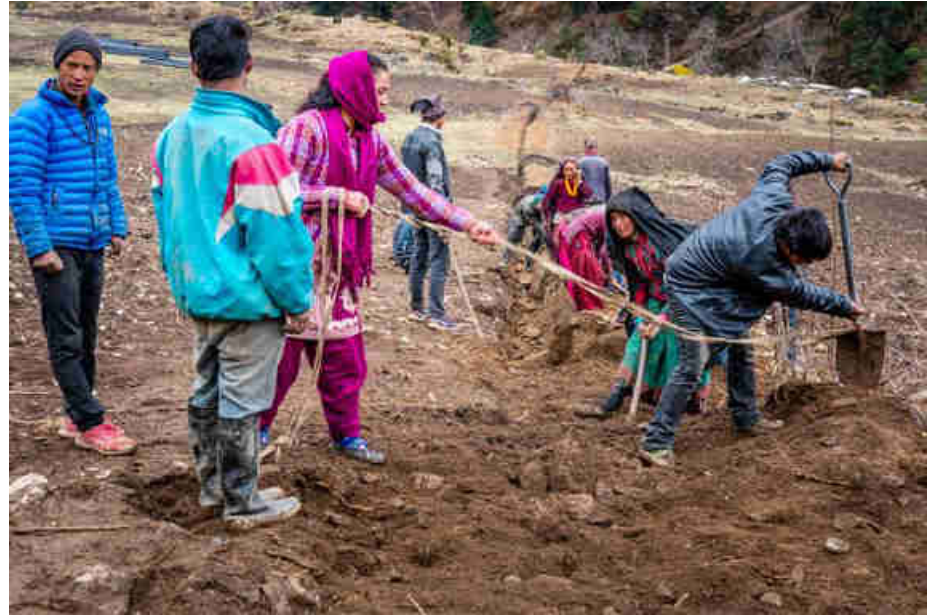
Pic. 32: Covering the power and communication cables with soil for protection
