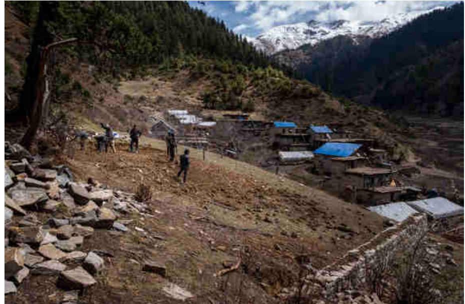
Pic. 100: Flatting the ground for the power house building structure
