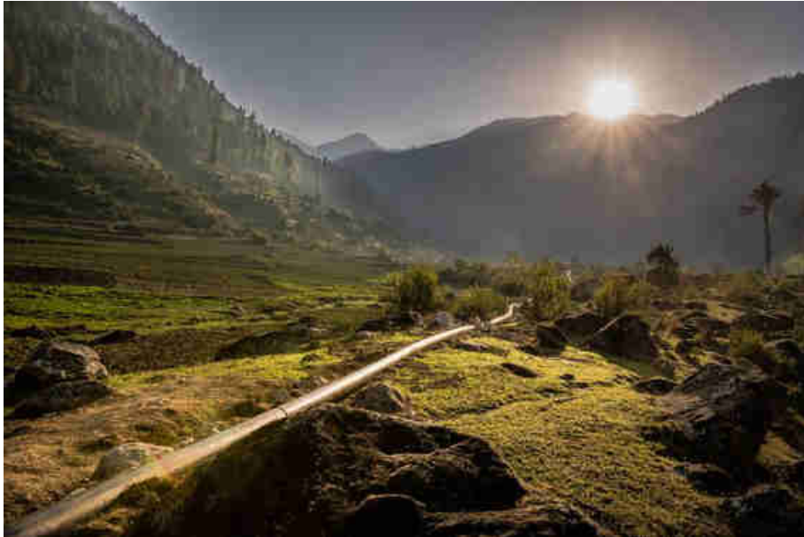
Pic. 75: The sun over the modular pico-hydro power penstock pipeline
