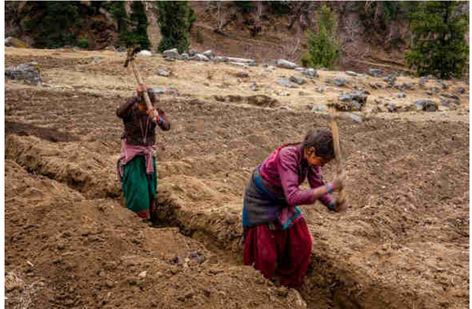
Pic. 20: Digging the canal for the underground power and communication cables
