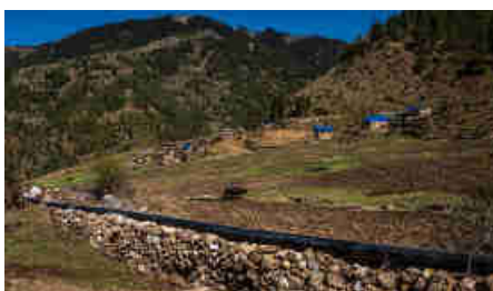
Fig. 4: Elevated Section of Penstock
