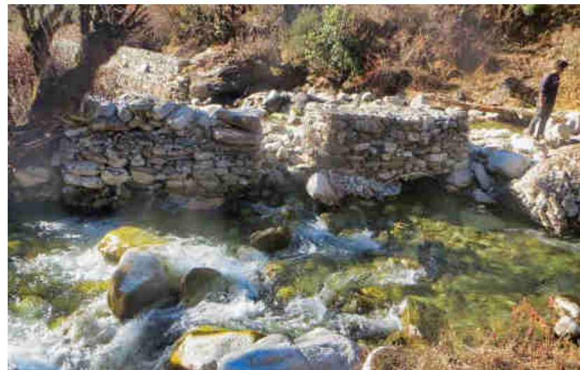
Pic. 2: Between the built stone walls flows the rushing river water into the created pond (pic. 3) to calm down and separate the gravel through gravity.
