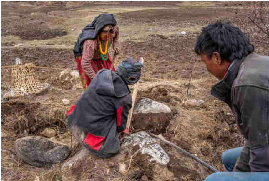
Pic. 13: Clearing the HDPE penstock pipeline path from large rocks
