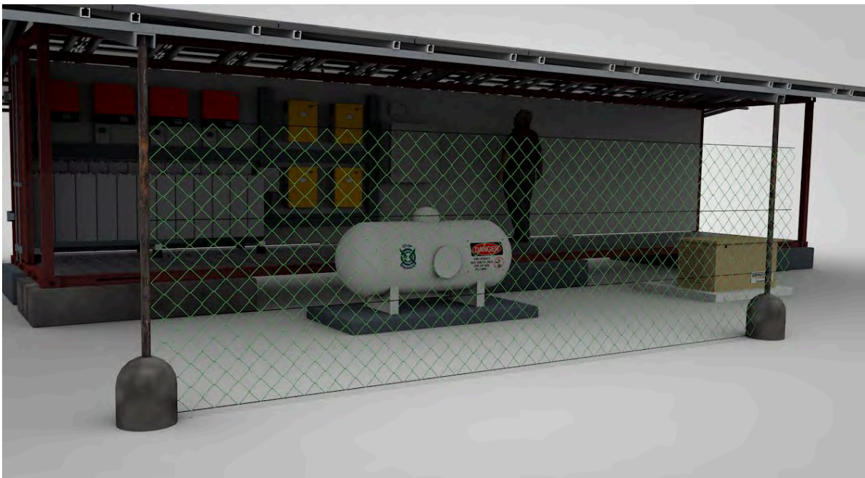
Picture 4: Gas-tank and LP-gas generator outside the container
