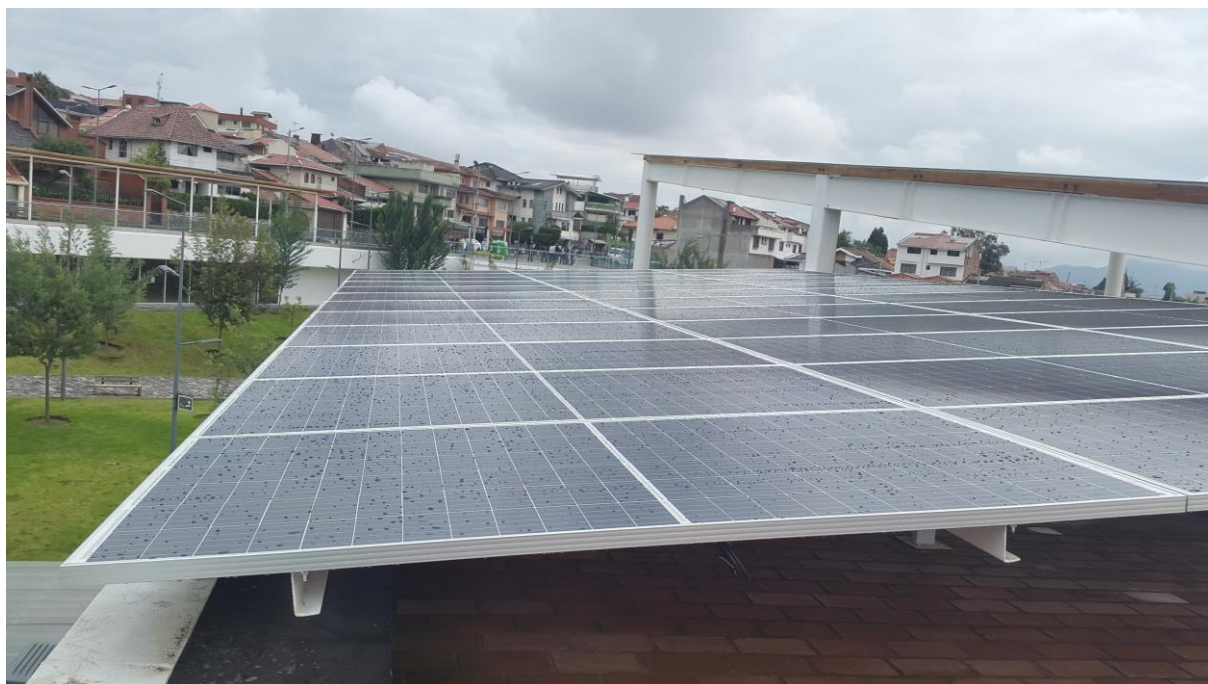
Figure 1: Solar system installation in Cuenca.
