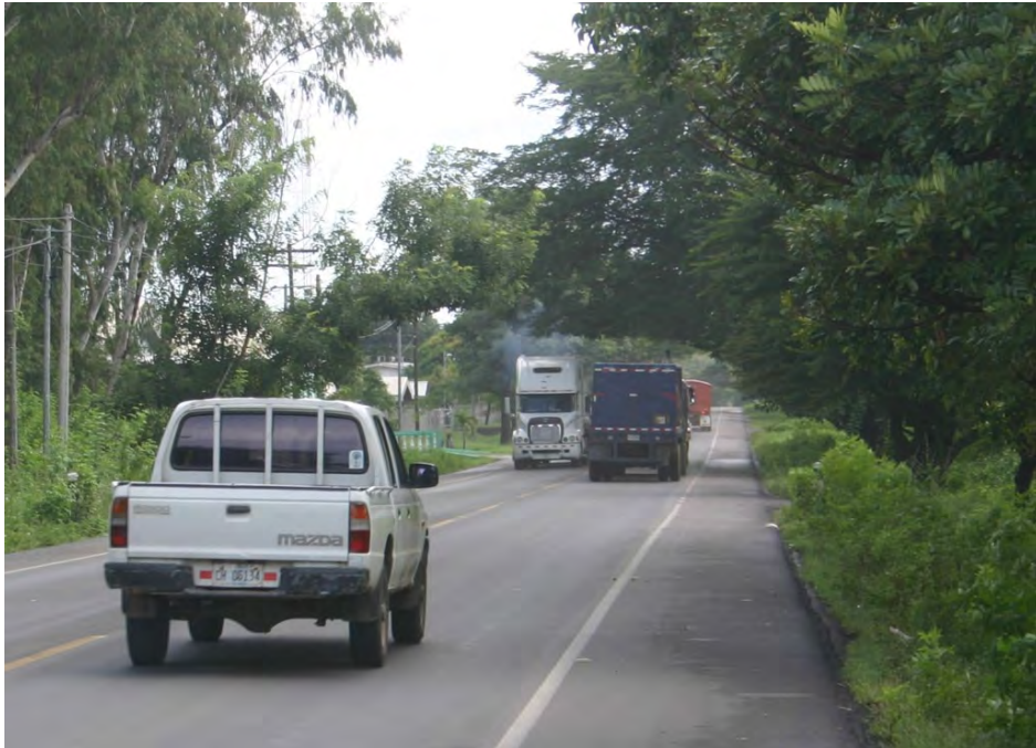
Figure 17: Tree branches can present obstacles in the range of 5–5.5 m (the white truck is approx. 4 m high).
