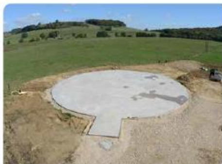
Day 1: Prefabricated slab by the client
