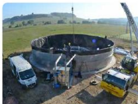
Day 3: Inner lining of the digester
