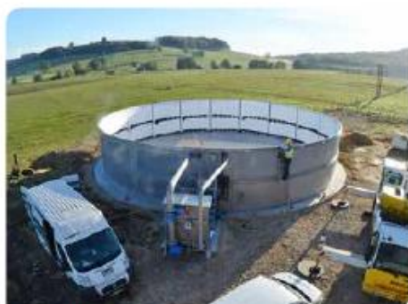
8:00 pm: Wall panels are assembled
