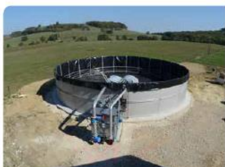
Day 4: Digester walls assembled
