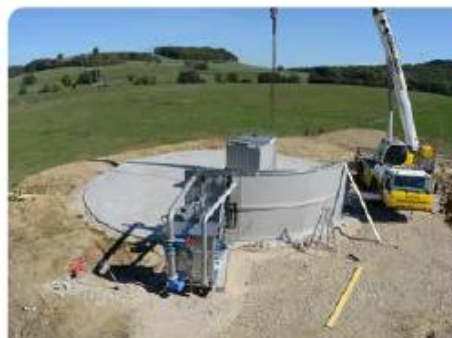
12:00 pm: Position of the technical module and first wall panels
