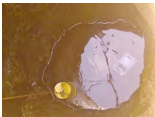
One of the unprotected wells in Funzi Island
