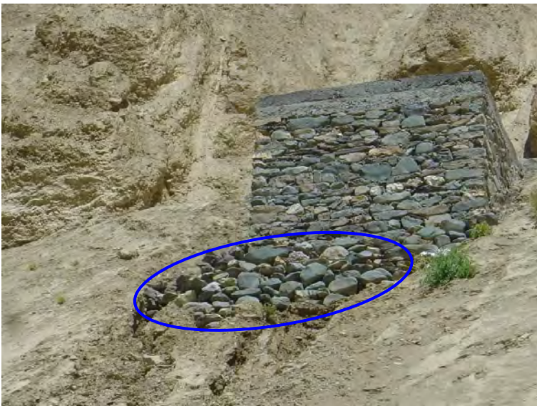
Picture 6.7 Temporary fixed forebay foundation
