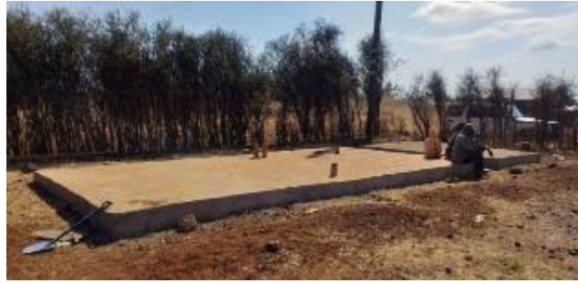
Figure 5. The cement slab realised
