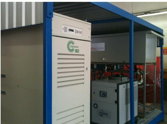
The "heart" of the plant: a 65 kW microturbine from Capstone.
